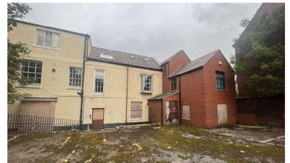
02. View of existing - Rear Elevation
