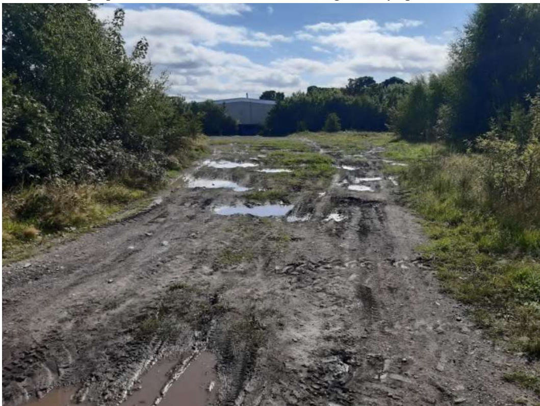
Photograph 8 Showing water ponding on site
