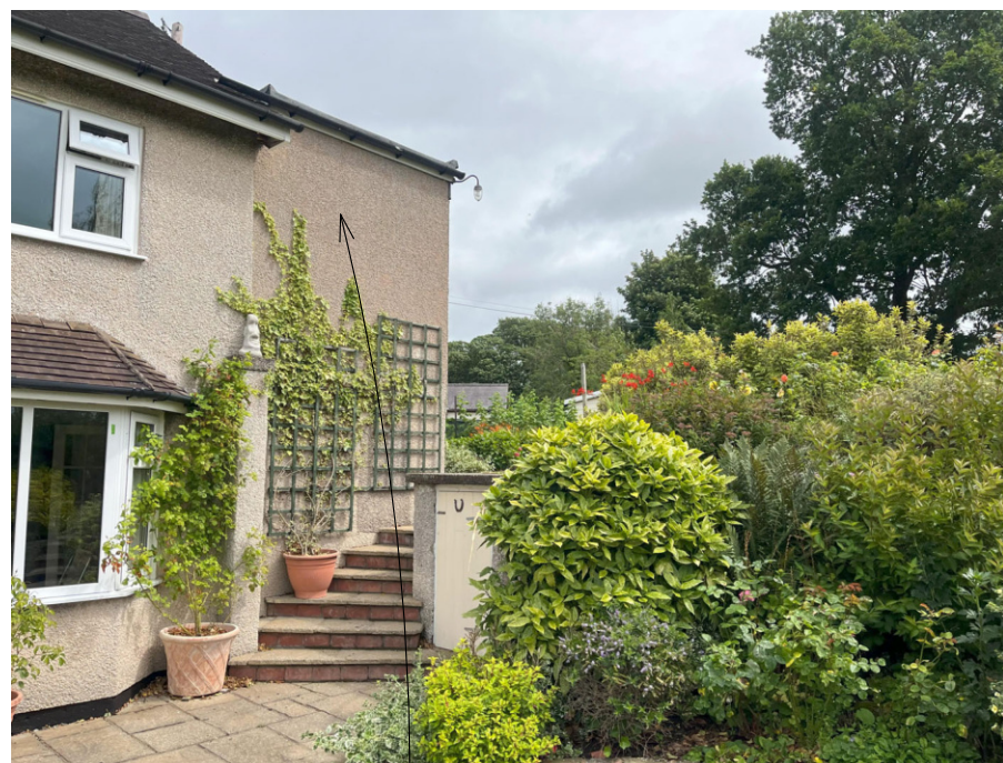
First floor dressing room to be demolished to first floor level (lower garden view)
