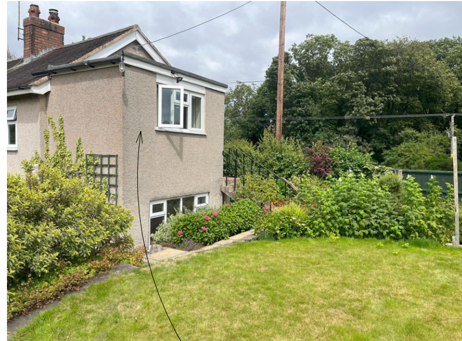
First floor dressing room to be demolished to first floor level (upper garden view)
