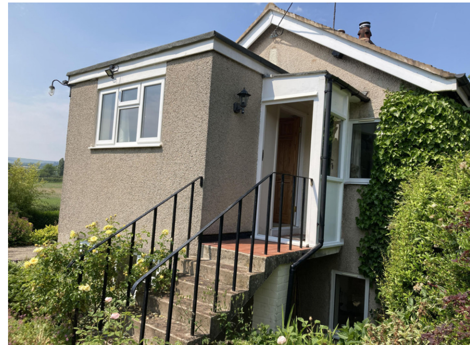
View of garden stair, landing and porch cantilevered over void below
