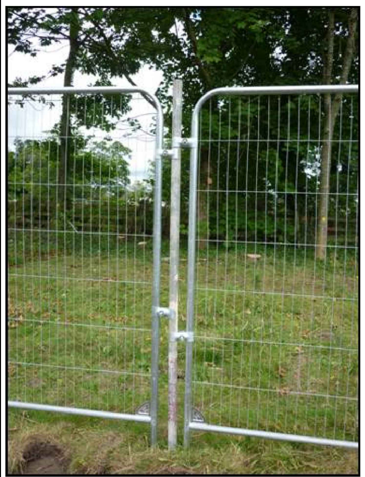
Tree Protective Fencing Specification
