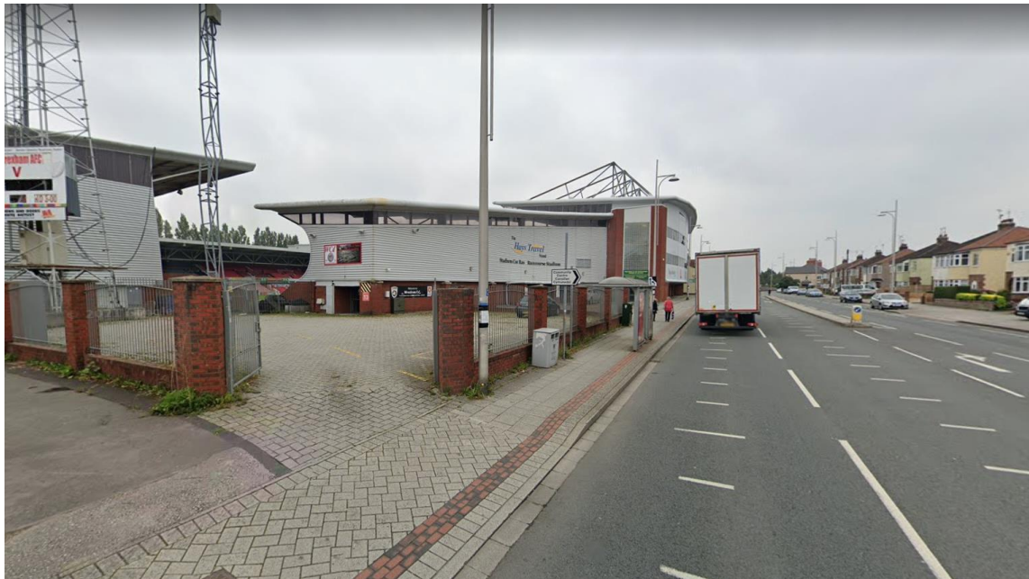
Figure 2.3: Existing dropped kerb access from Mold Road
