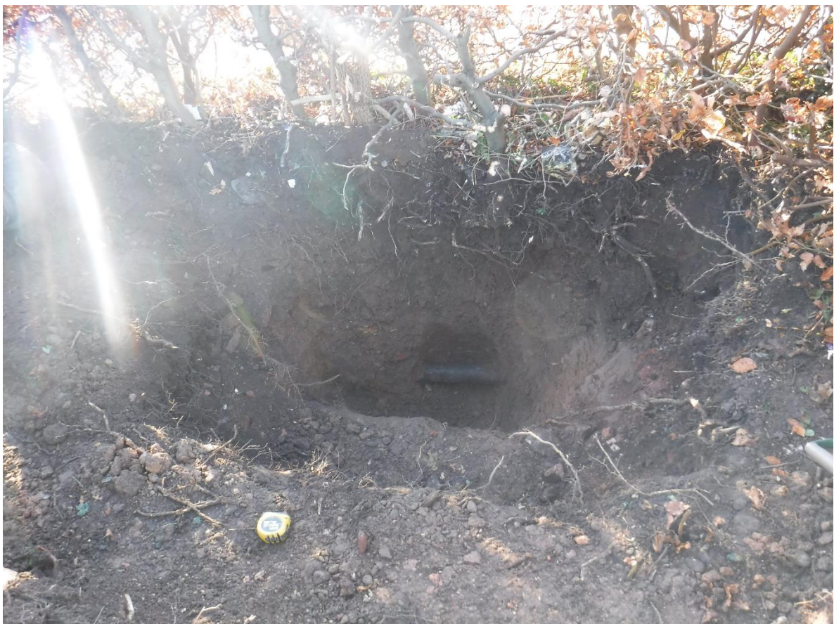
Access point excavated on rising main 3rd excavation in hedge line
