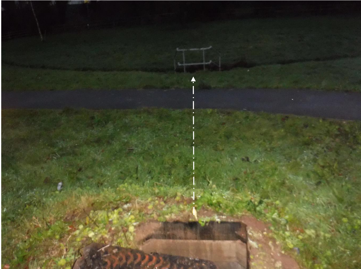
Generic No MH15 discharging to outfall at watercourse
