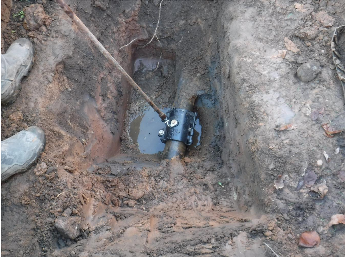
Access point repaired on rising main 2 nd excavation & back filled
