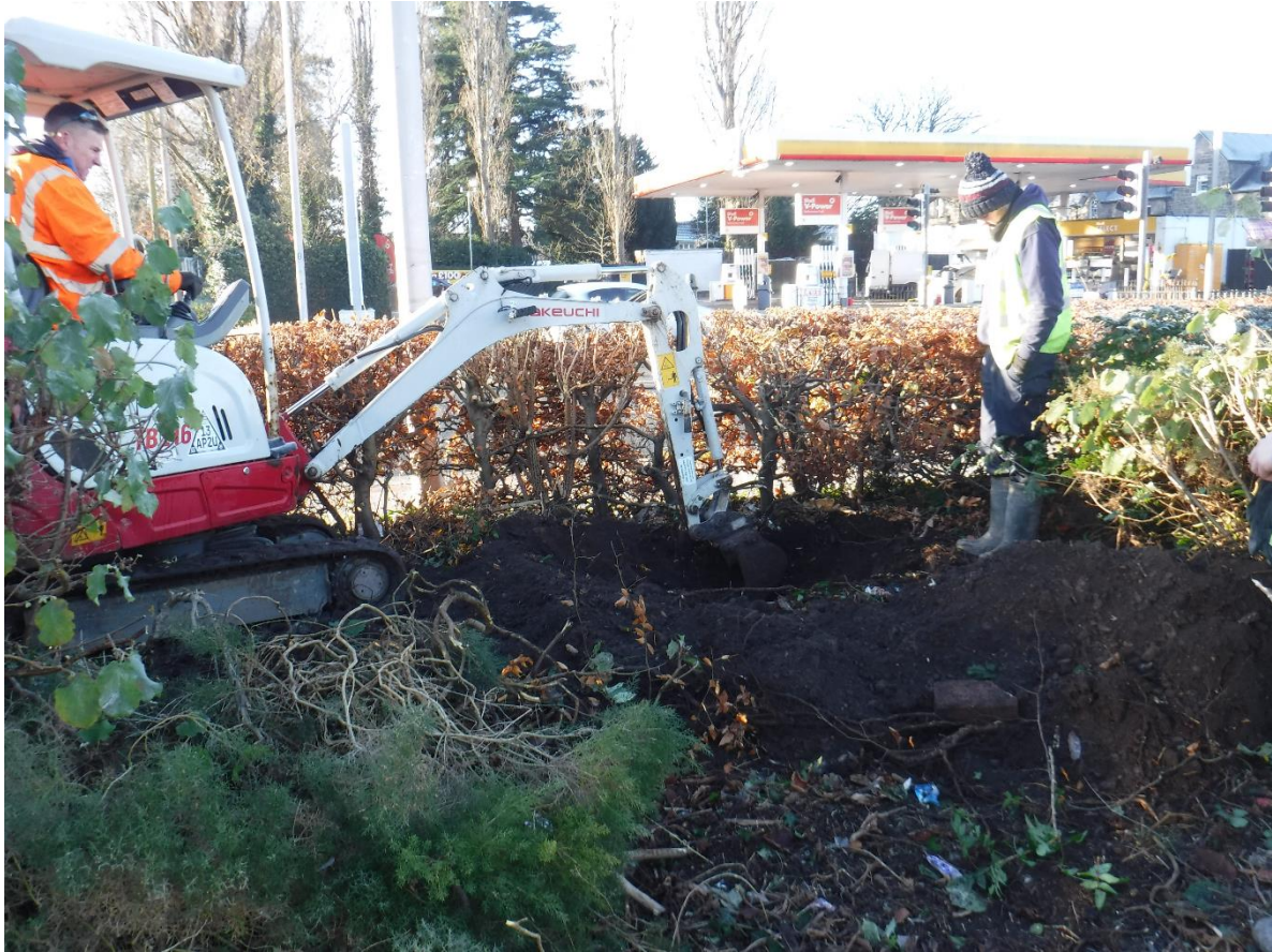
Access point excavated on rising main 3rd excavation in hedge line
