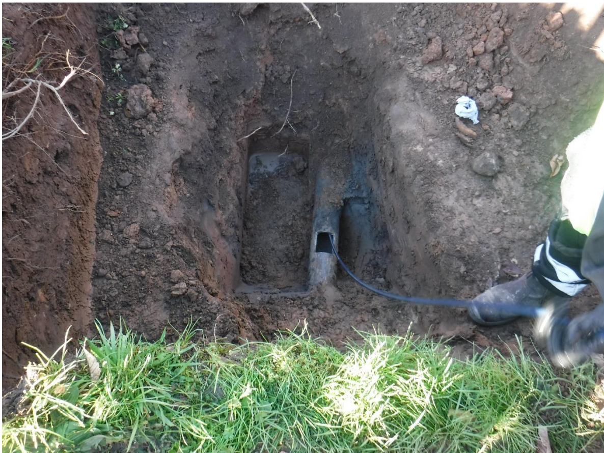
2 nd Excavation adjacent to main entrance gateway – access point on rising main
