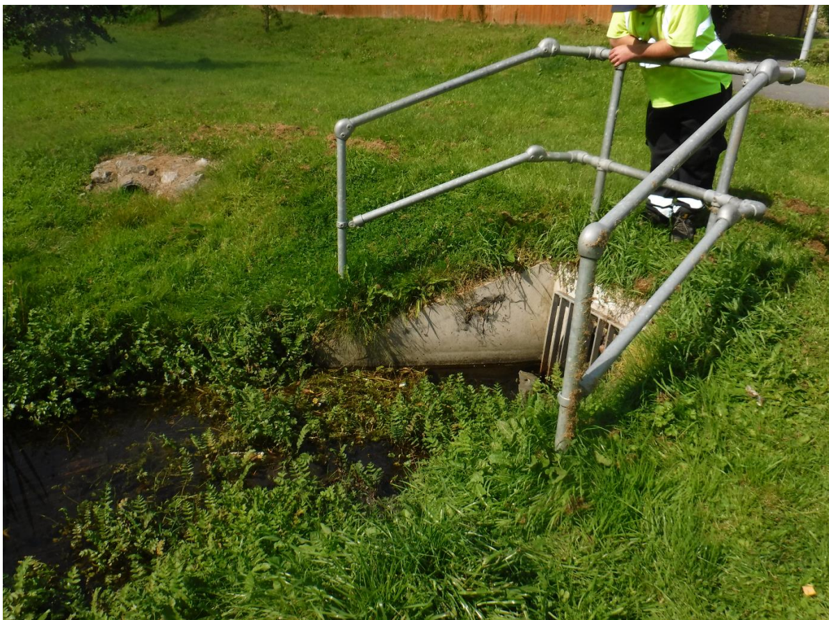
Generic No MH15 discharging to outfall at watercourse
