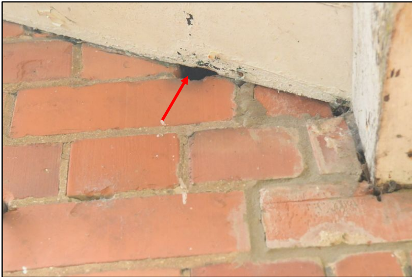
Small brickwork gap
