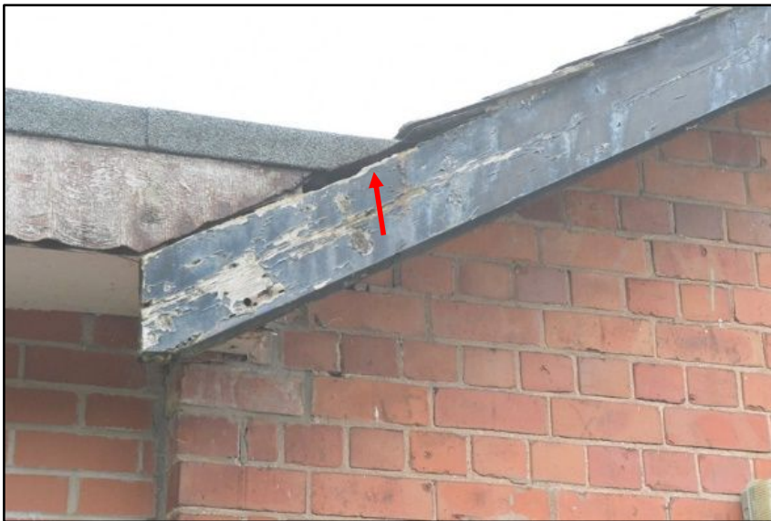
Gap between flat roof and slate, the same on the other side as well
