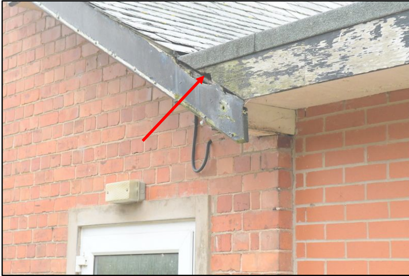
Small brickwork gap
