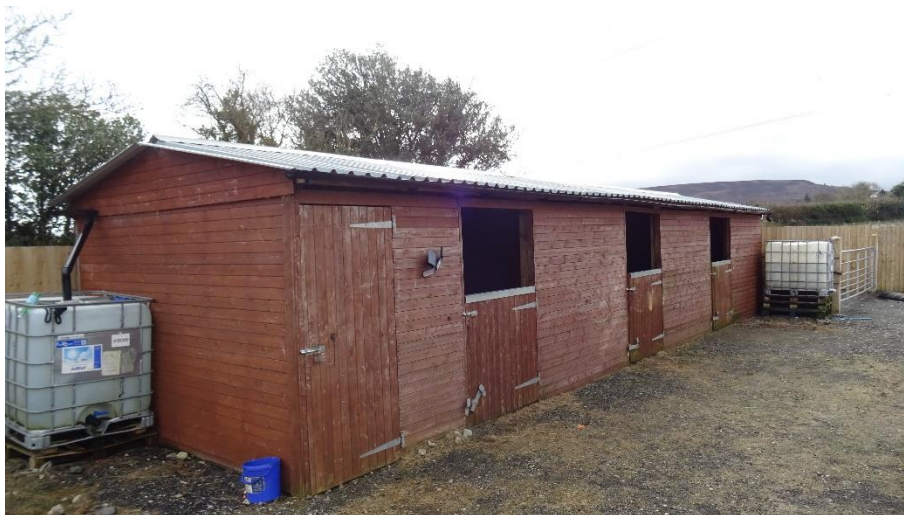
Figure 4.3. Larger stable building
