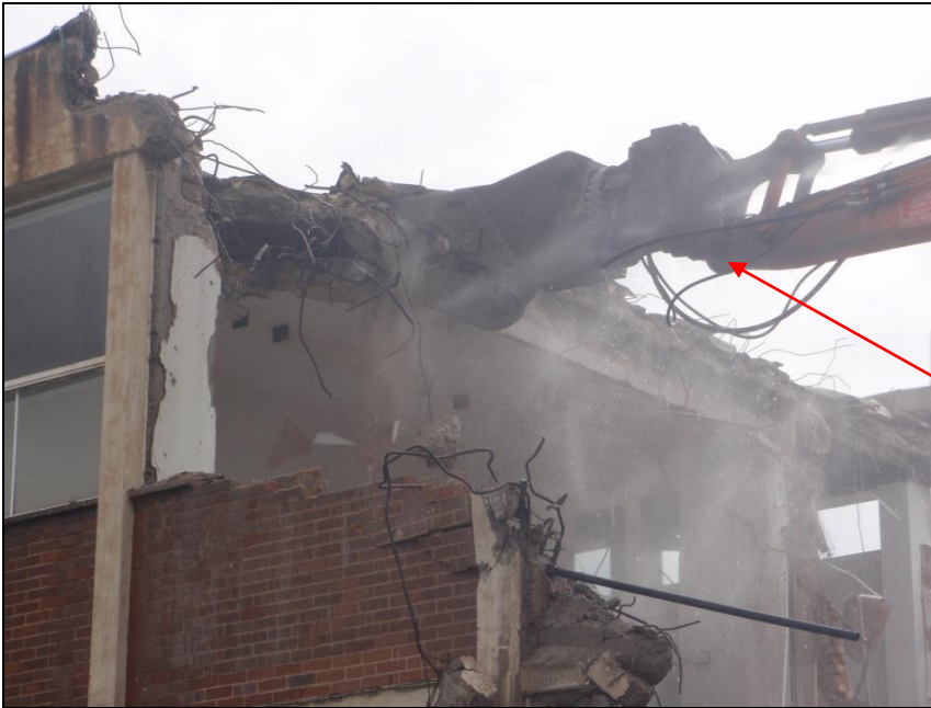
Dust suppression at source
