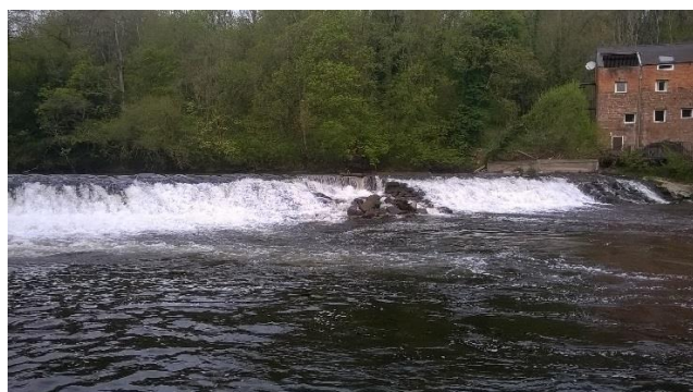
Plate 8-28. Poor condition of the weir including the collapsed section, looking from the RHB downstream of the weir
