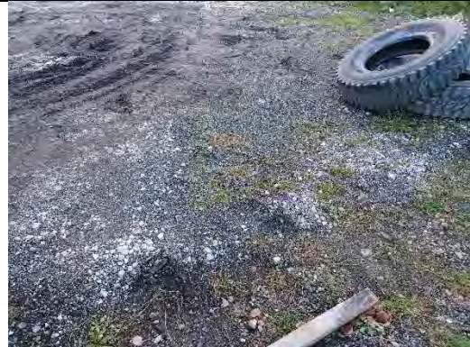
Close up view of the hardstanding / gravelled site surface.
