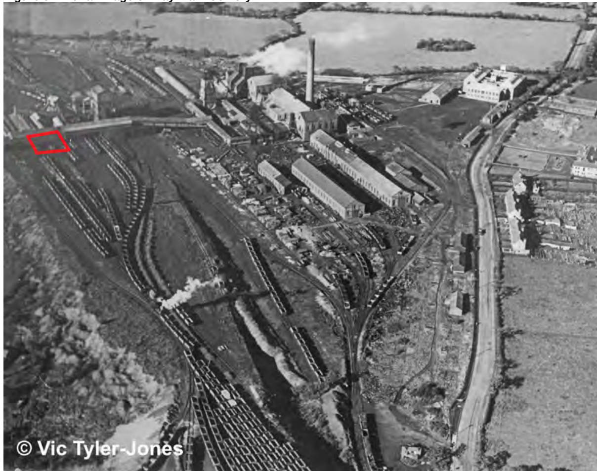
Figure 5.2 Aerial image of Llay Main Colliery 7
