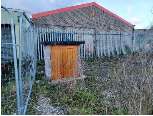
View of the service box (potentially electrical) which lies to the east of the site.
