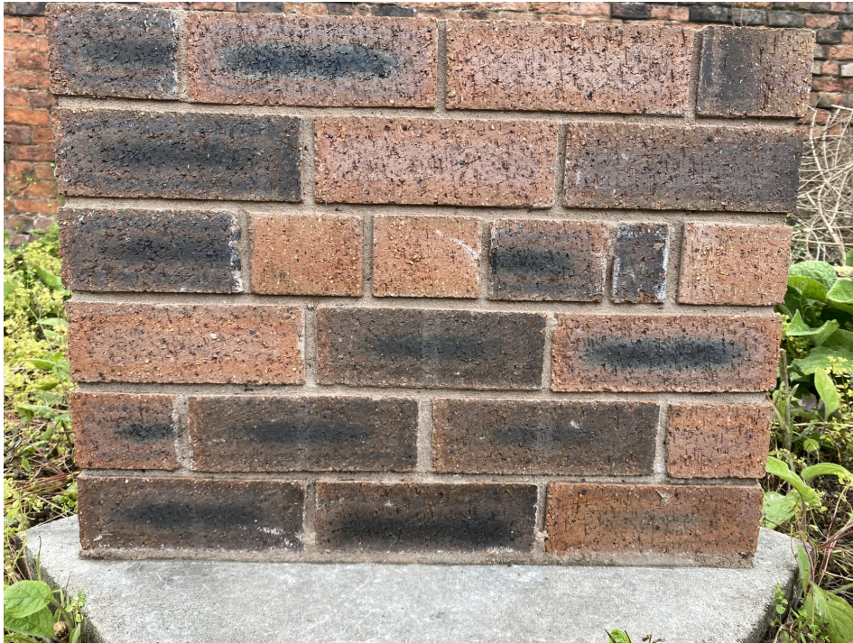
Sample mortar mix for wall with approved Snowie Heritage 73mm Dragwire brick . Mortar mix = 1 part Hanson NHL 3.5 hydraulic Lime 3 parts coarse sand from Borrás quarry.
