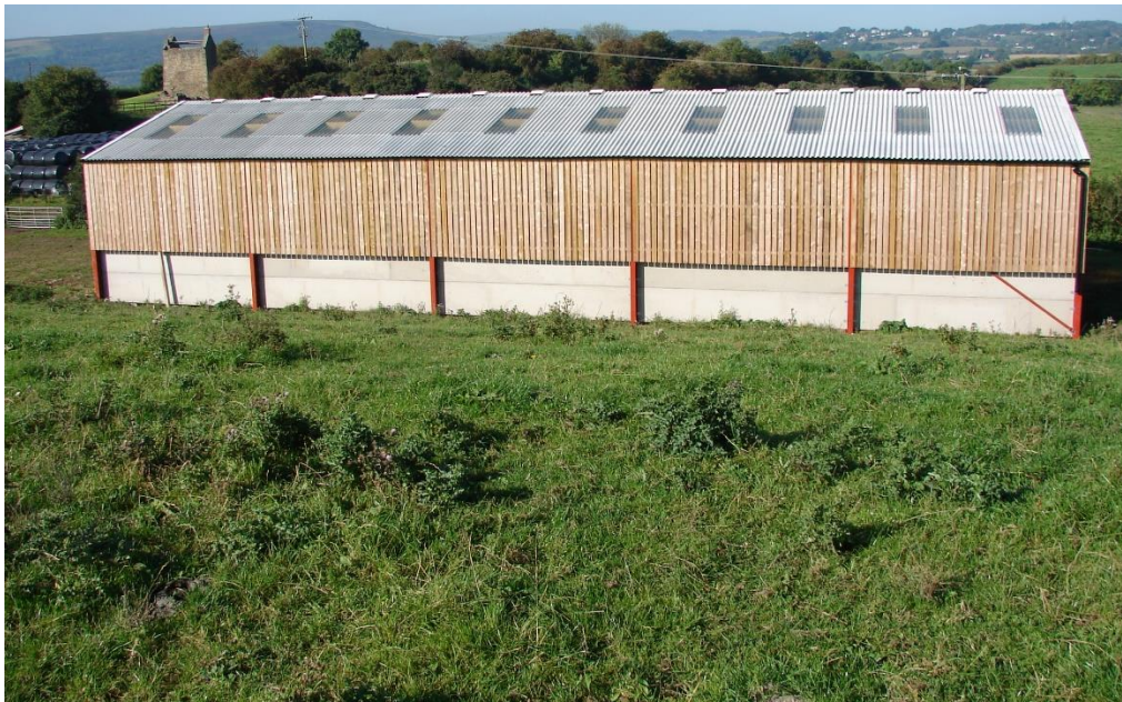
View of the building from the east.
