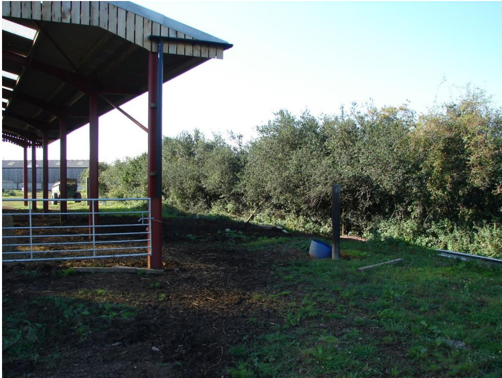
The hedge to the west of the building.
