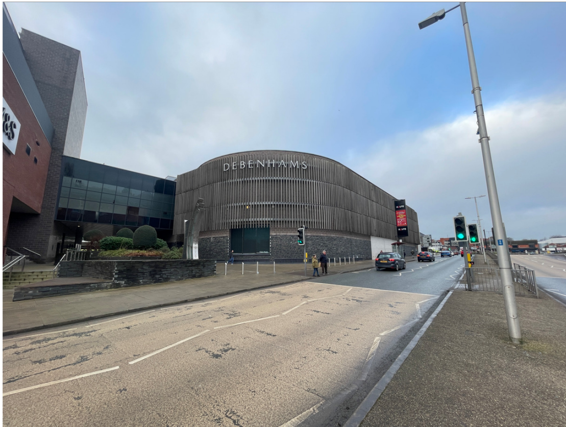
Photo 3 – Zetland Street, as existing
