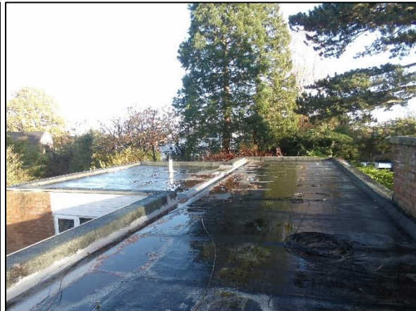
Figure 4: The roof of the building.
