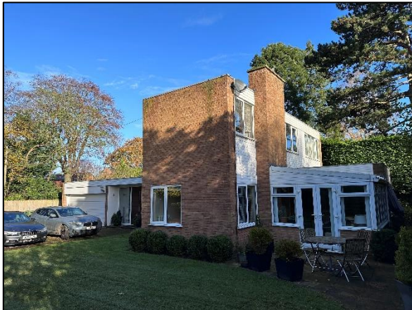
Figure 3: The building viewed from the southwest.
