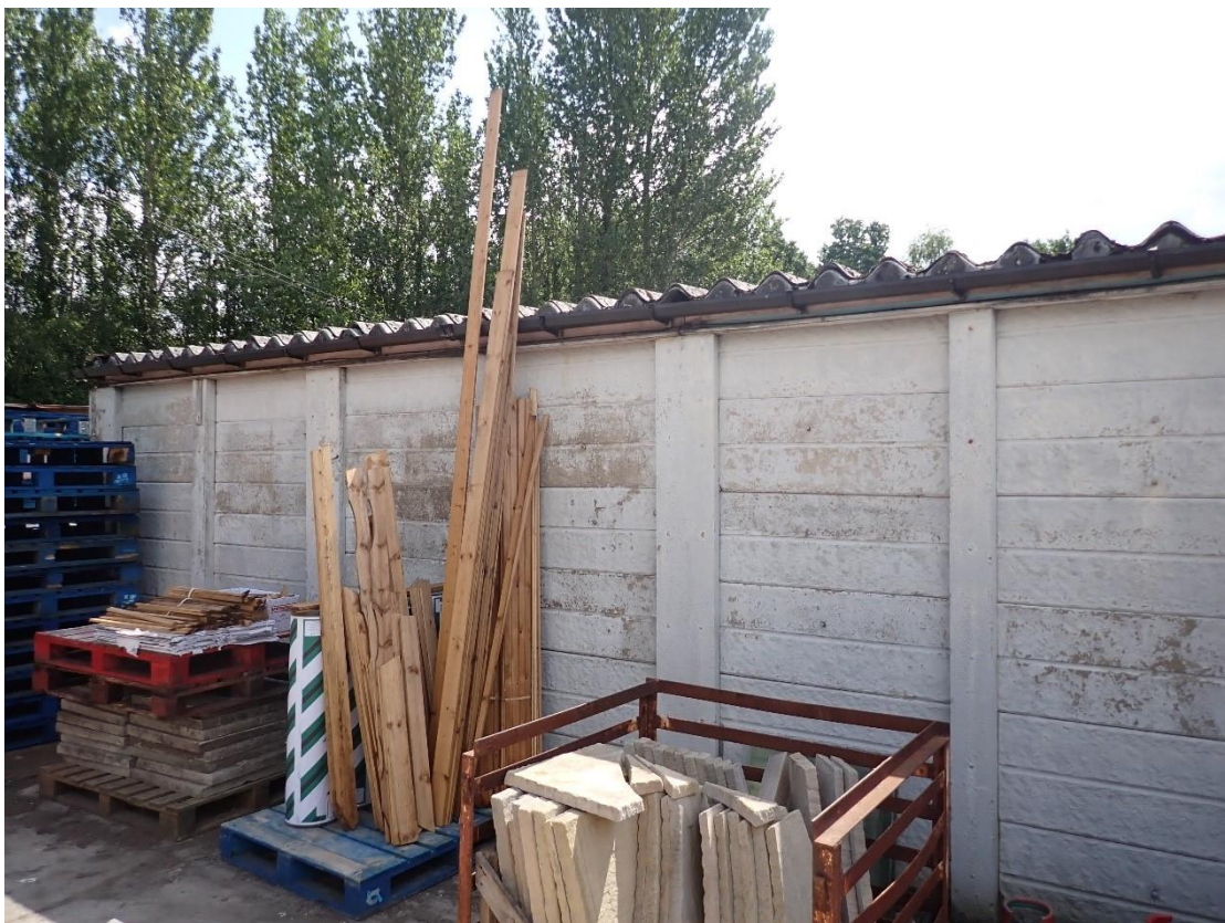
Photograph 10. The northwestern aspect of Building 2.
