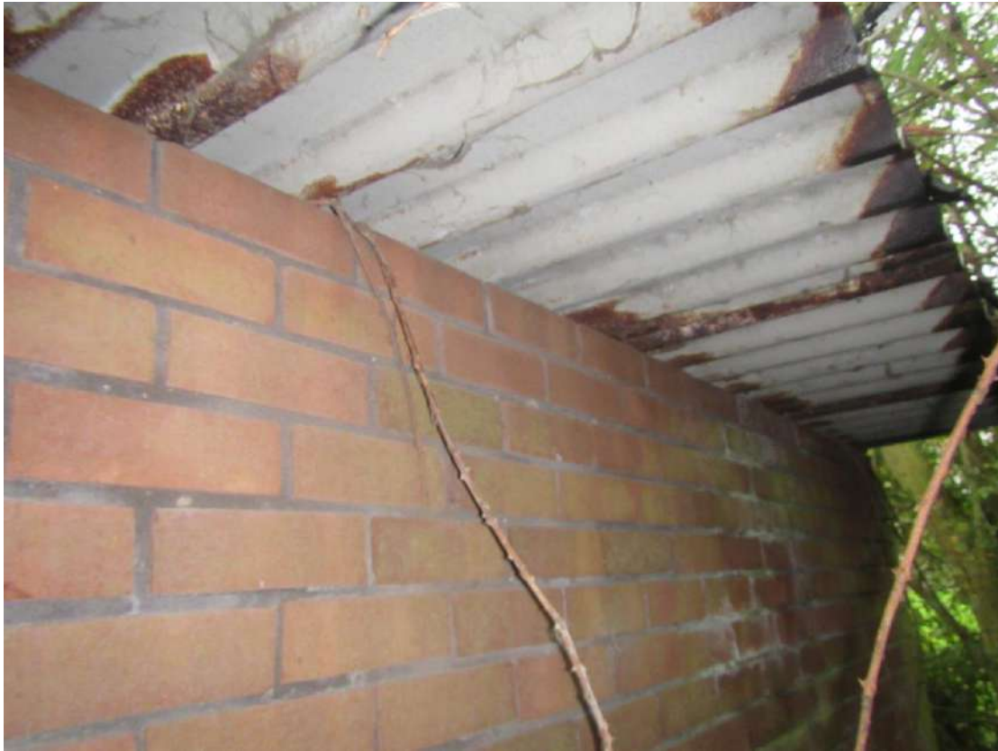
Photograph 7. The structure of the roof and external walls of the building adjacent to the site.
