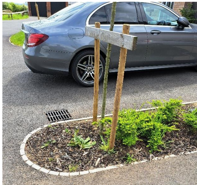
Figure 3 Poor planting practices to avoid: Restricted rooting volumes, impermeable surfacing and planting trees near underground services/drainage runs
