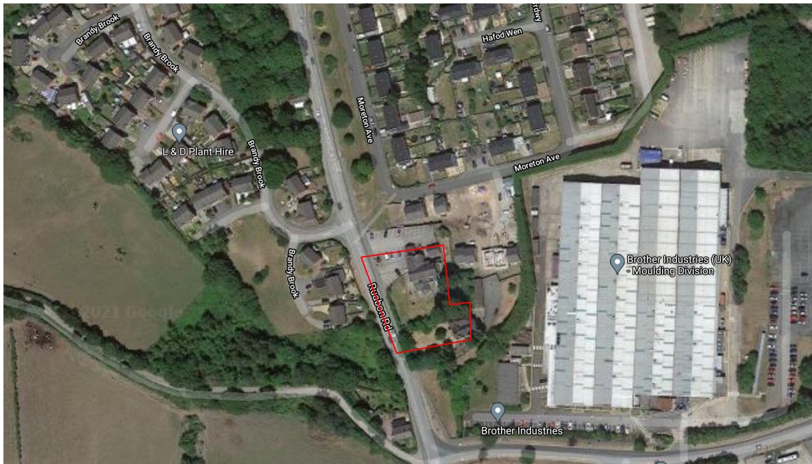
1. Satellite image of the site (Prior to demolition).
