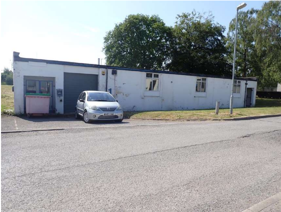
Photograph 5 – Northwestern aspect of Building 2.
