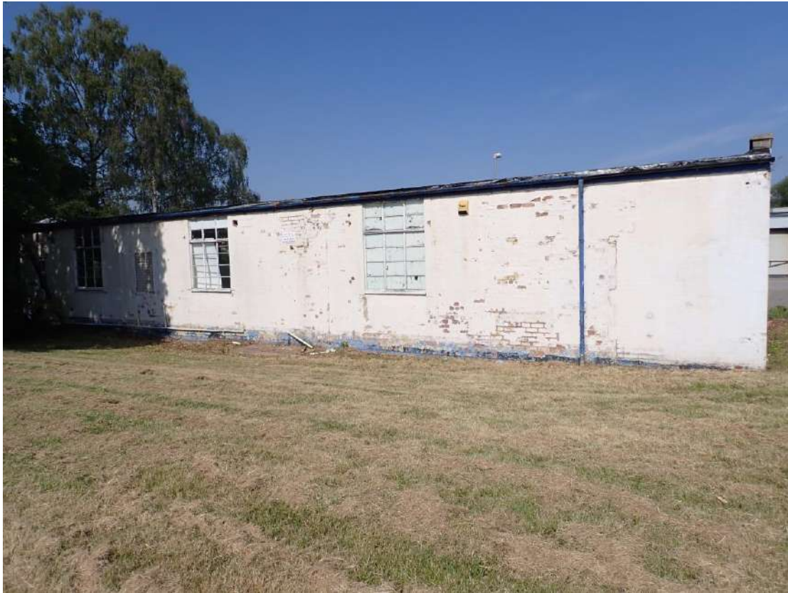
Photograph 7 – Southeastern aspect of Building 2.
