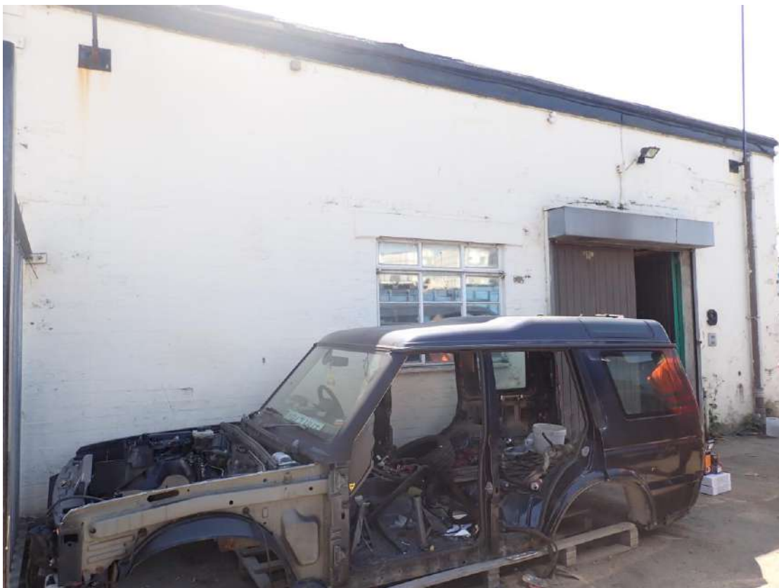
Photograph 24 – Northwestern aspect of Building 5.
