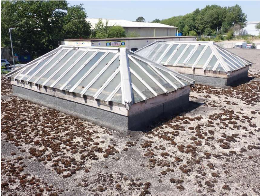
Photograph 19 - Roof of Building 4.
