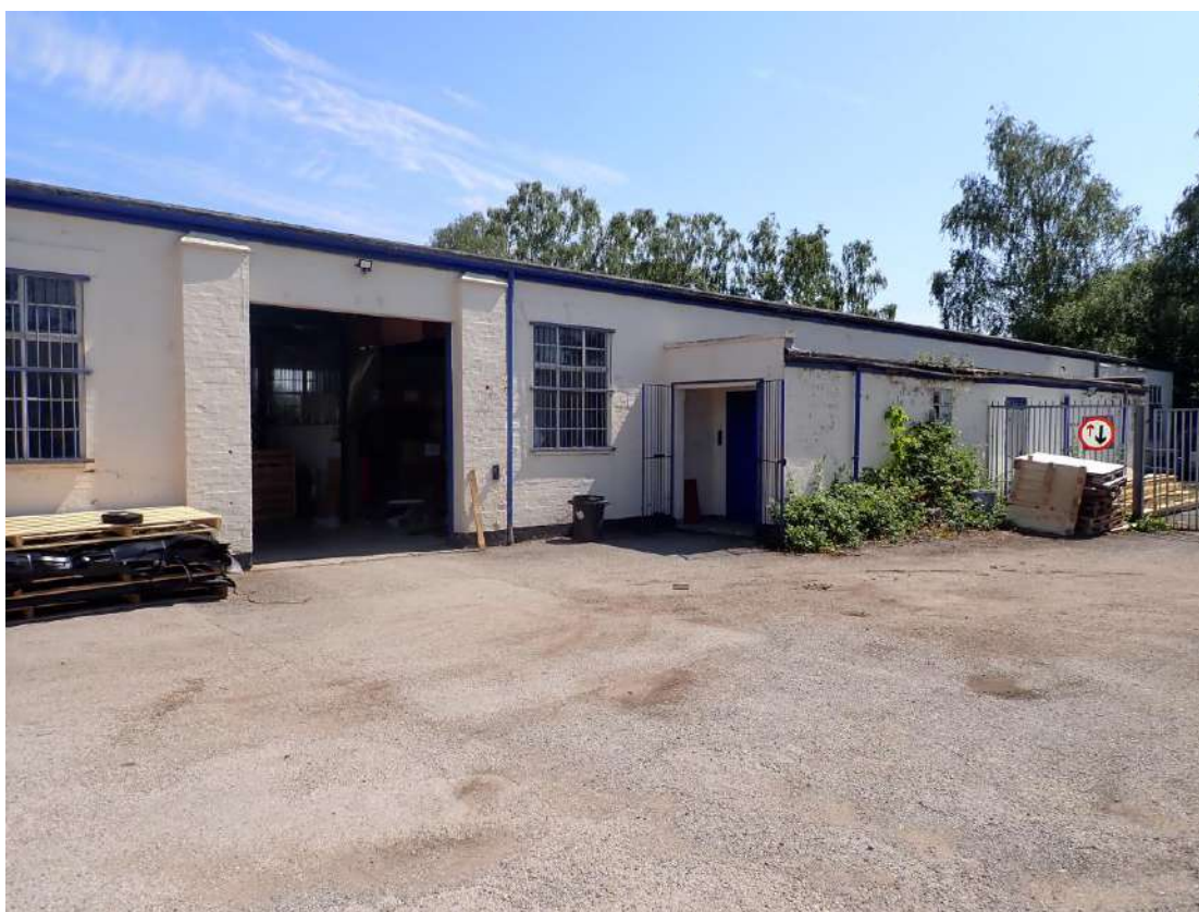
Photograph 14 – Southwestern aspect of Building 4.
