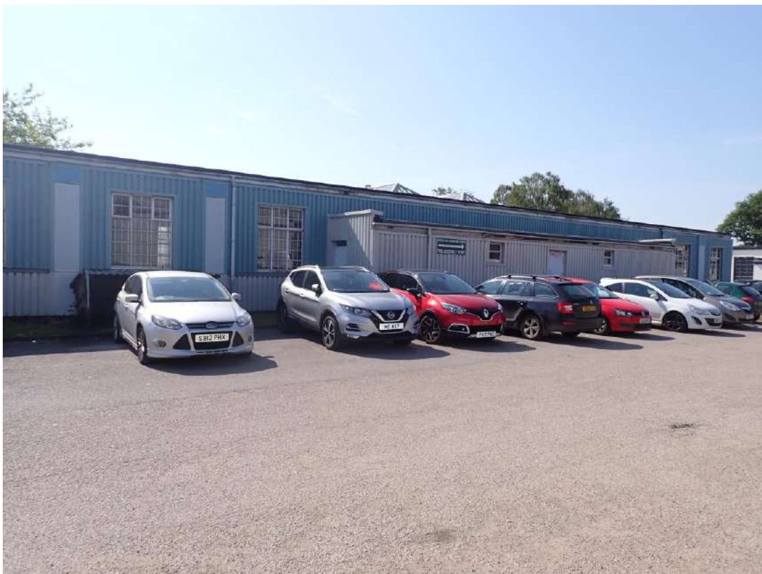
Photograph 4 – Northwestern aspect of Building 1.
