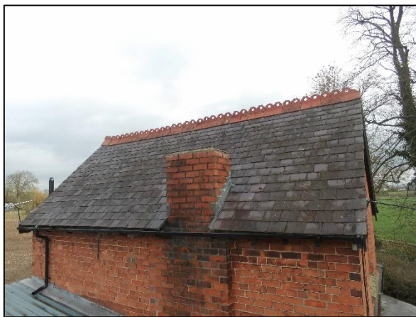
Figure 9: The roof and leadwork to the southwest.
