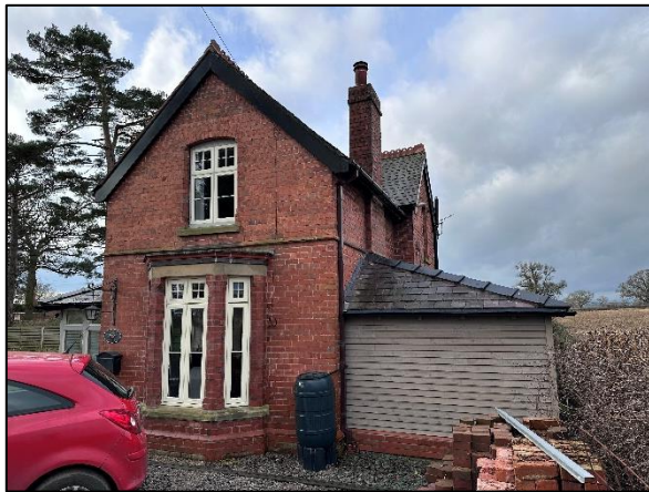
Figure 3: The northeast elevation of the building.
