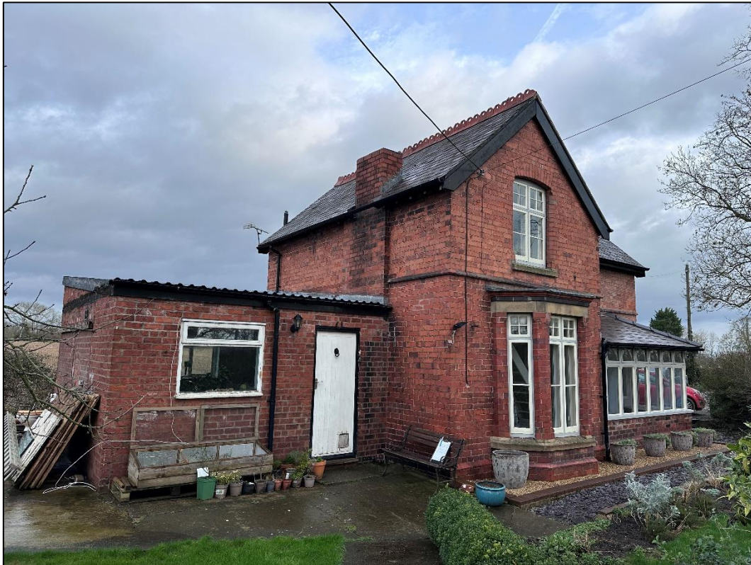
Figure 2: The southeast elevation of the building.
