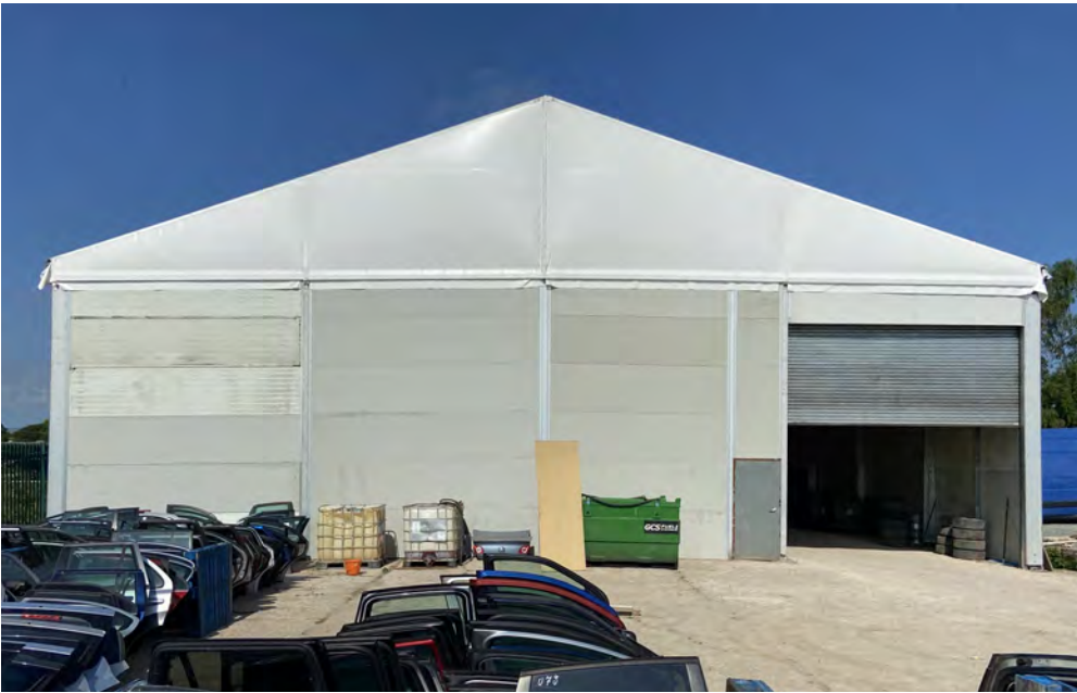
1. Building A - Front elevation as viewed from the East
