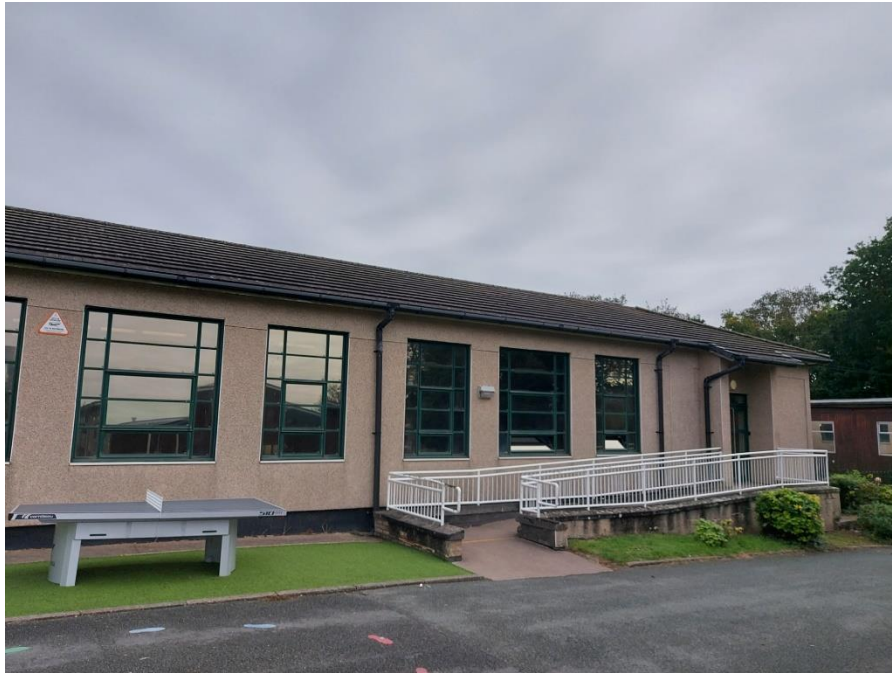
Single-storey school building at Target Note 9 .
