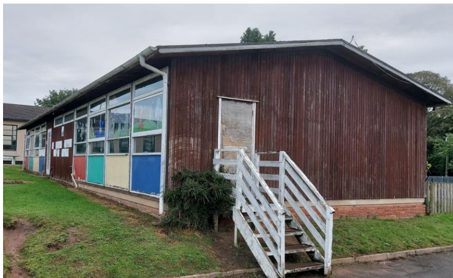
Building to be demolished at Target Note 1 .
