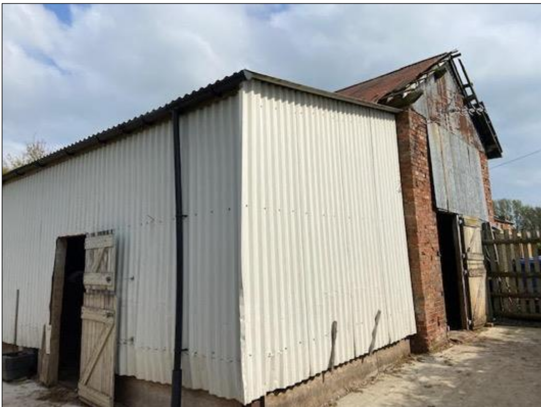
Photograph 4; A view of the corrugated extension section of the building.
