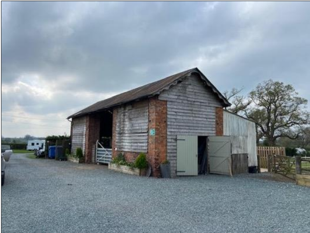
Photograph 1; A view of the subject building. The large openings across the building can clearly be seen.
