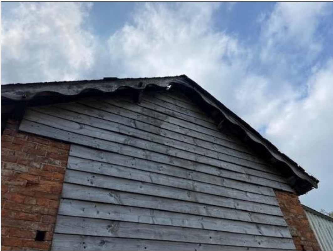
Photograph 2; A view of the northern face of the building. The gable comprises wooden paneling and wooden soffit boarding.
