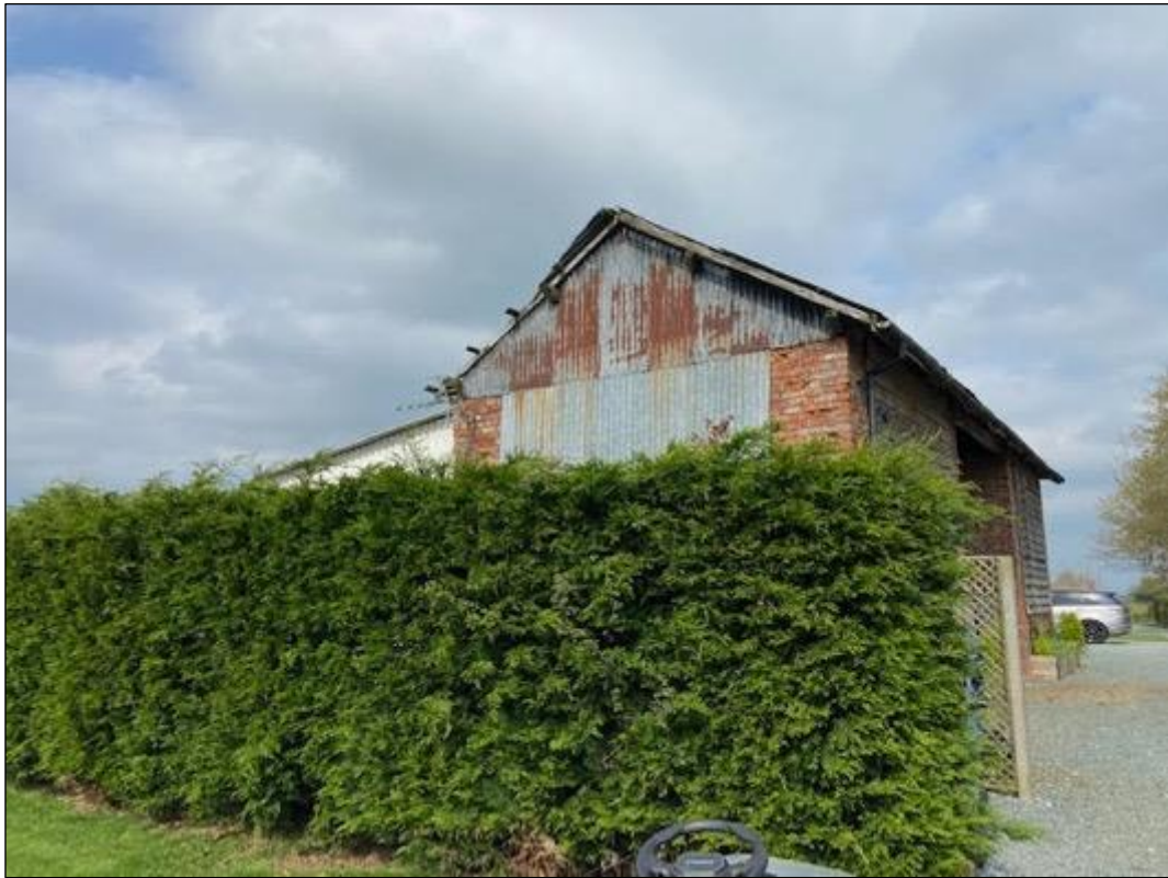
Photograph 7; Corrugated tin external upper walls and roof feature on the building.
