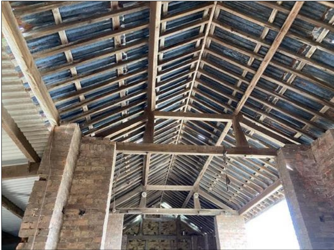
Photograph 5; An internal view of the subject building; wooden purlins and rafters support the corrugated tin external roof.
