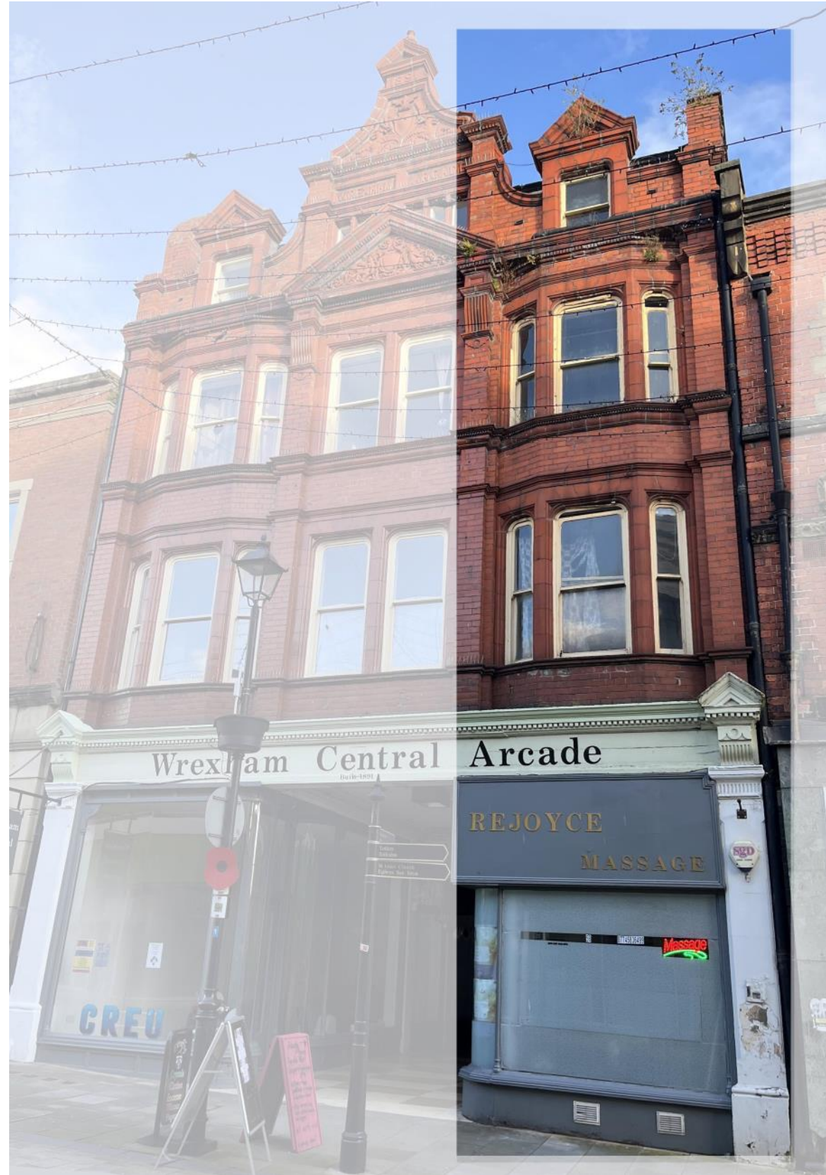
Image 01 - Photograph of existing front elevation with No. 58 highlighted
