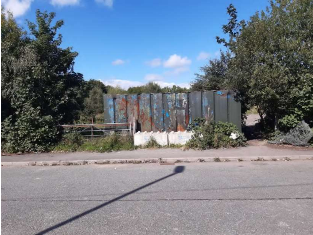
Photograph 5 Site access on southern site boundary
