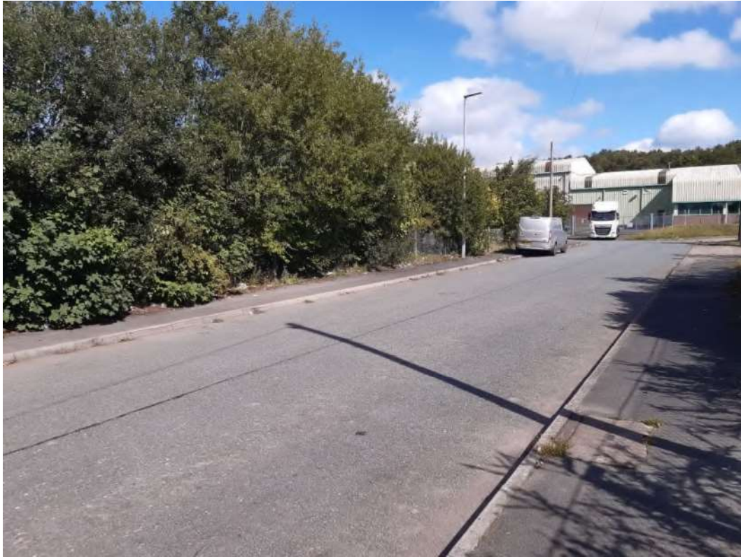
Photograph 3 Southern boundary road
