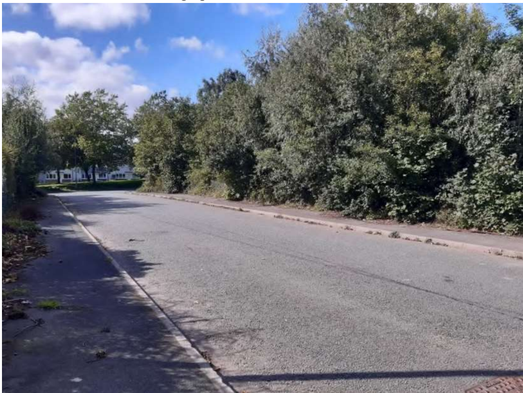
Photograph 4 As above looking west
