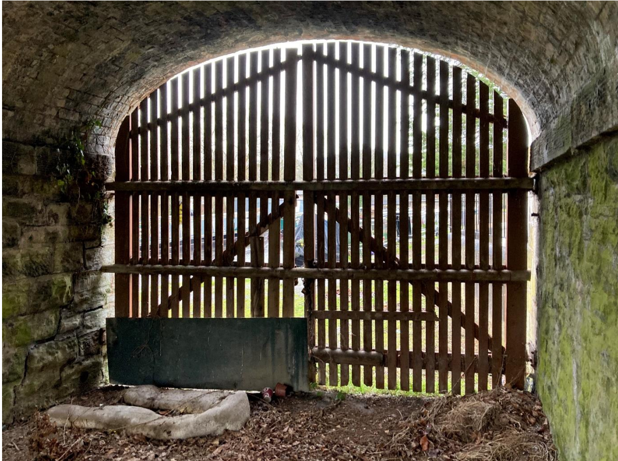
Figure 5: Existing security gate on the south facing elevation of the western aperture.
