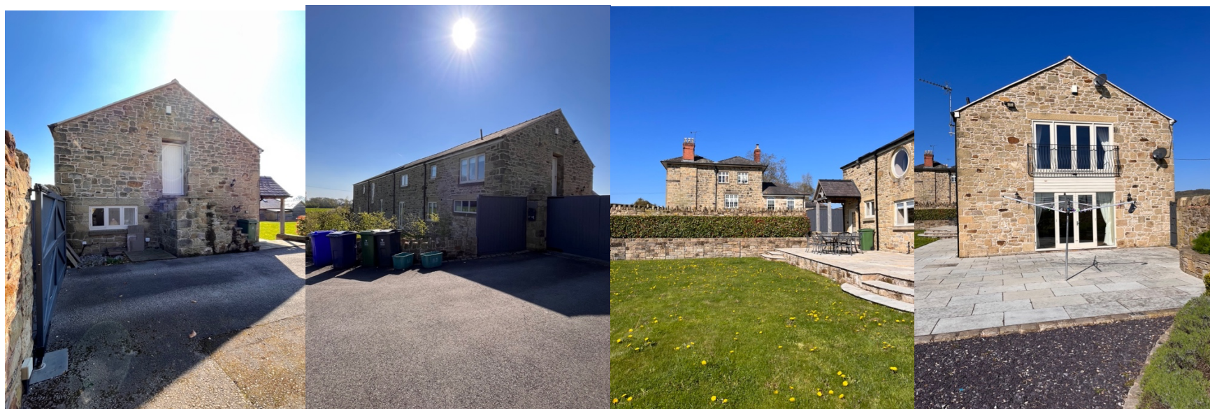
Fig 6. The barn. From left to right: The west gable, the rear north elevation facing the road, the farmhouse east gable facing the courtyard, with the front elevation of the truncated barn just visible; and the barn's east gable. Note domestic openings to the gable end –full length French doors to ground and first floor and Juliet balcony.
