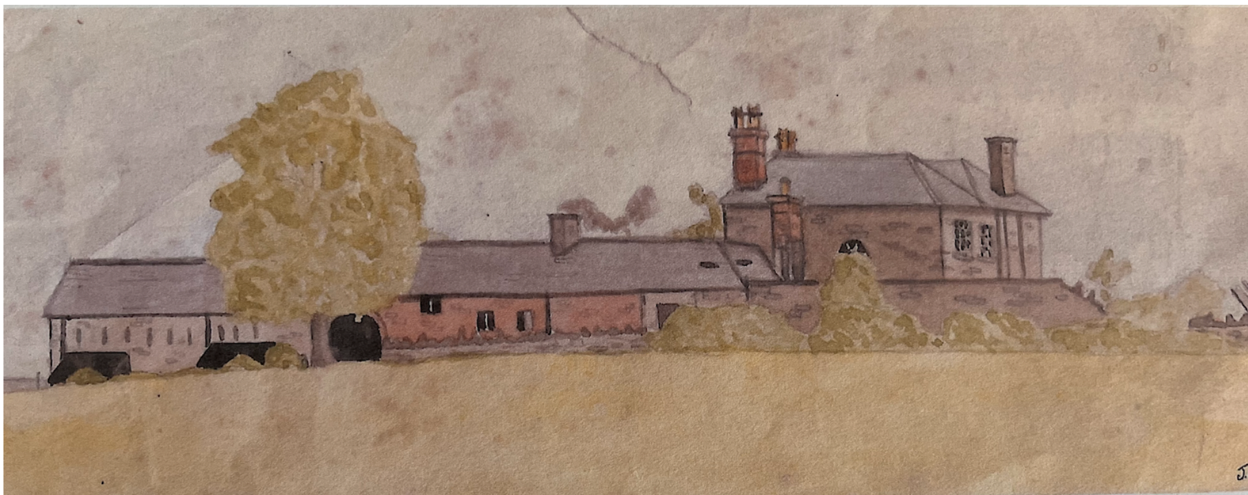
Fig 4. A watercolour, showing the house to the right with the attached farm buildings to the left. The barn that remains today now is on the far left of the tree. The remainder, from the cartshed opening to the house, was demolished in the 20 th century.
