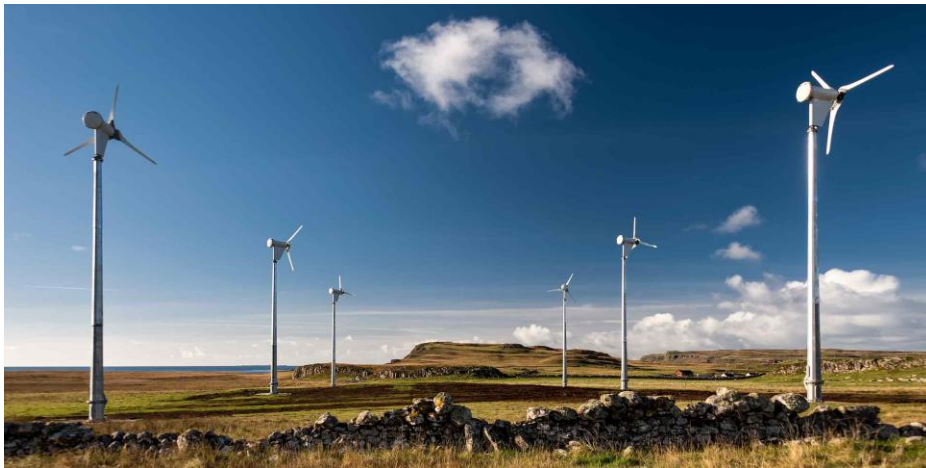
Figure 4 Typical 6kW Wind Turbine Example
