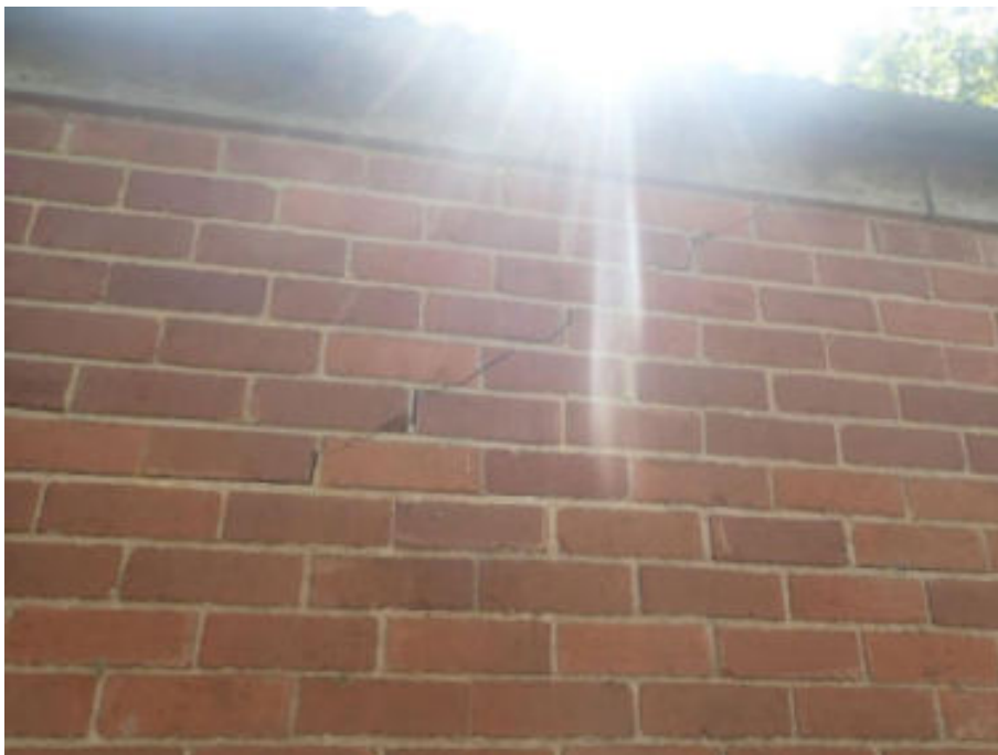
Figure 219. Diagonal fracture
