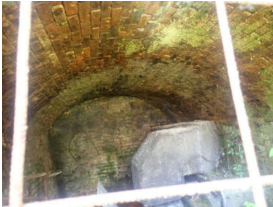
Figure 209. Deteriorated masonry
