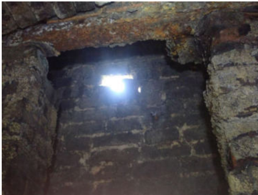
Figure 182. Corroded lintel
