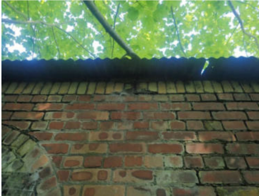
Figure 6. Typical de-bonded brick coping
