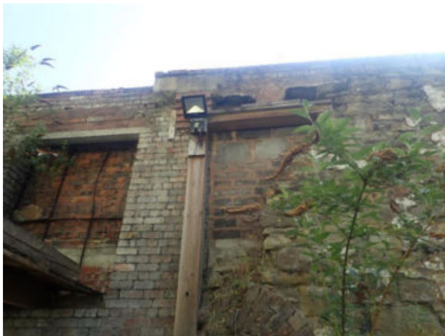
Figure 148. Temporary timber propping
