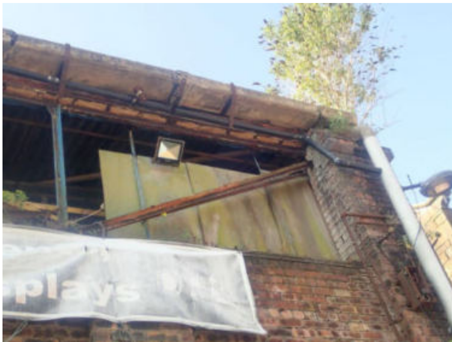
Figure 52. Sheared angle
