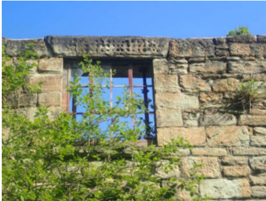
Figure 59. Typical failed stone jam
