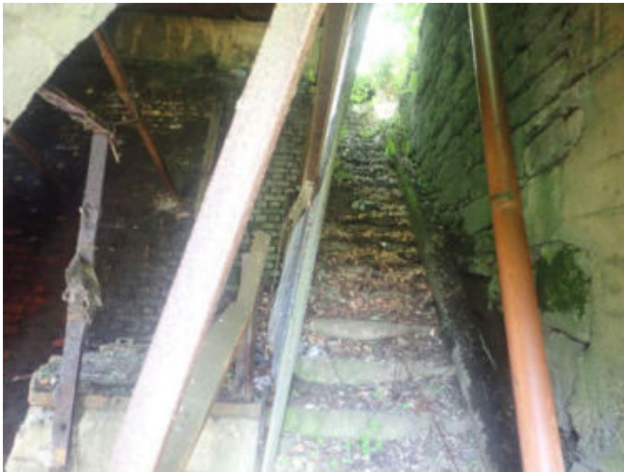
Figure 194. Deteriorated frame
