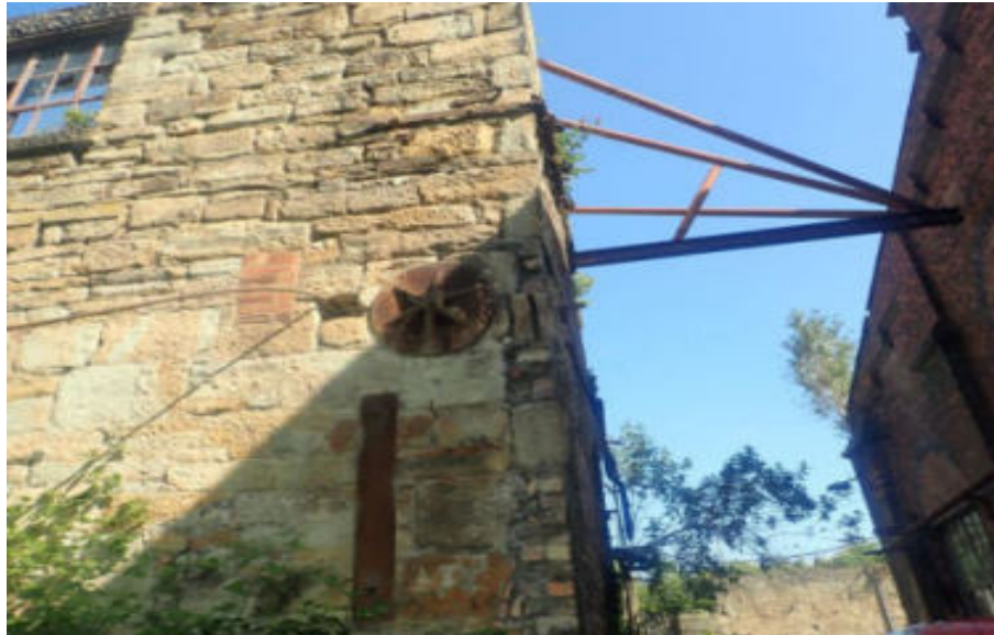
Figure 70. Steel prop
