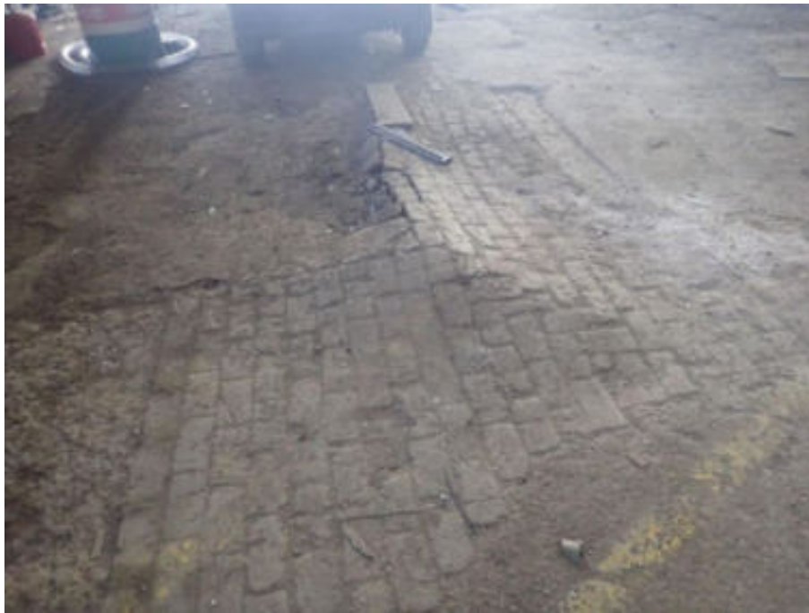
Figure 57. Deformed floor
