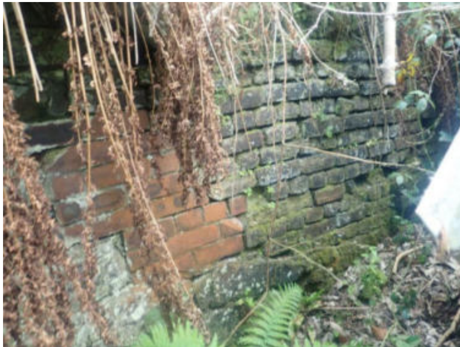
Figure 109. Historic brick repair
