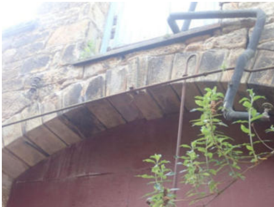
Figure 58. Dropped arch
