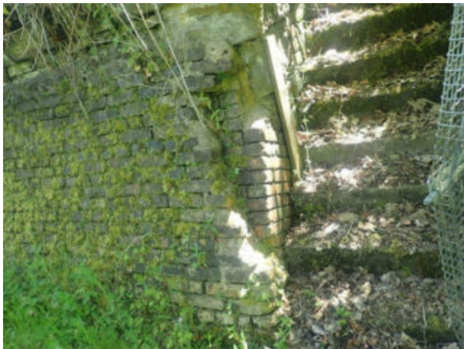
Figure 121. Missing masonry
