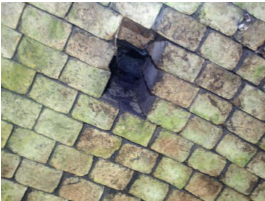
Figure 186. Dislodged bricks
