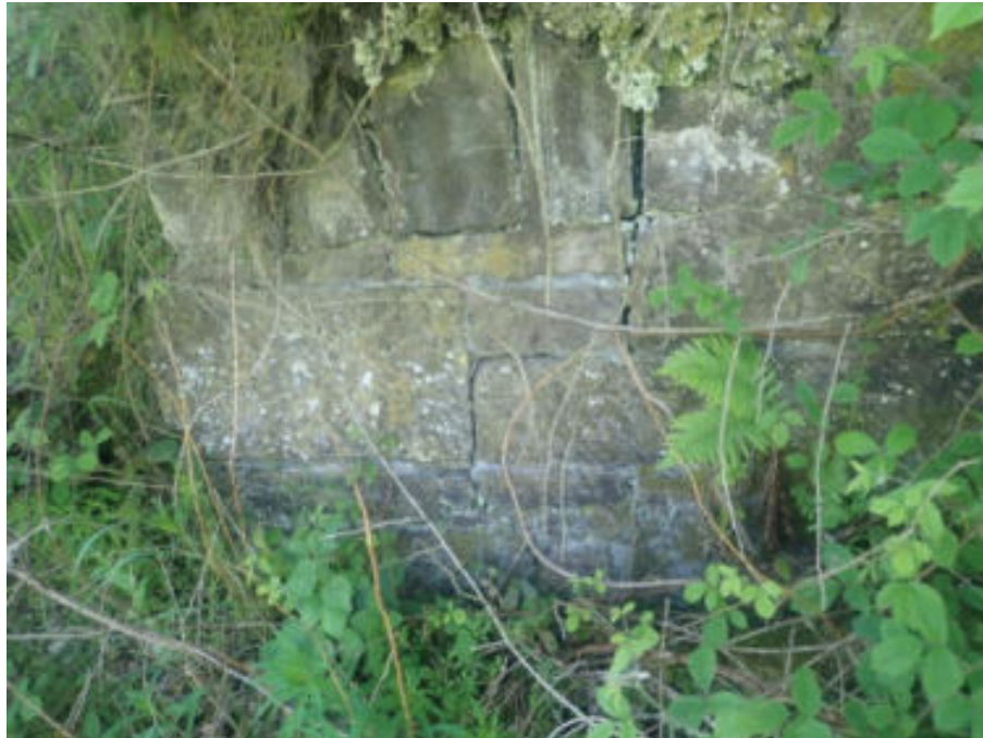
Figure 114. Diagonal fracture
