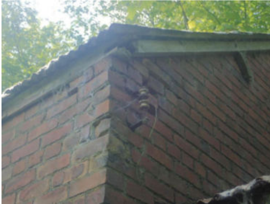
Figure 14. Loose/dislodged masonry
