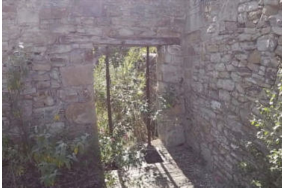
Figure 68. Propped timber lintel
