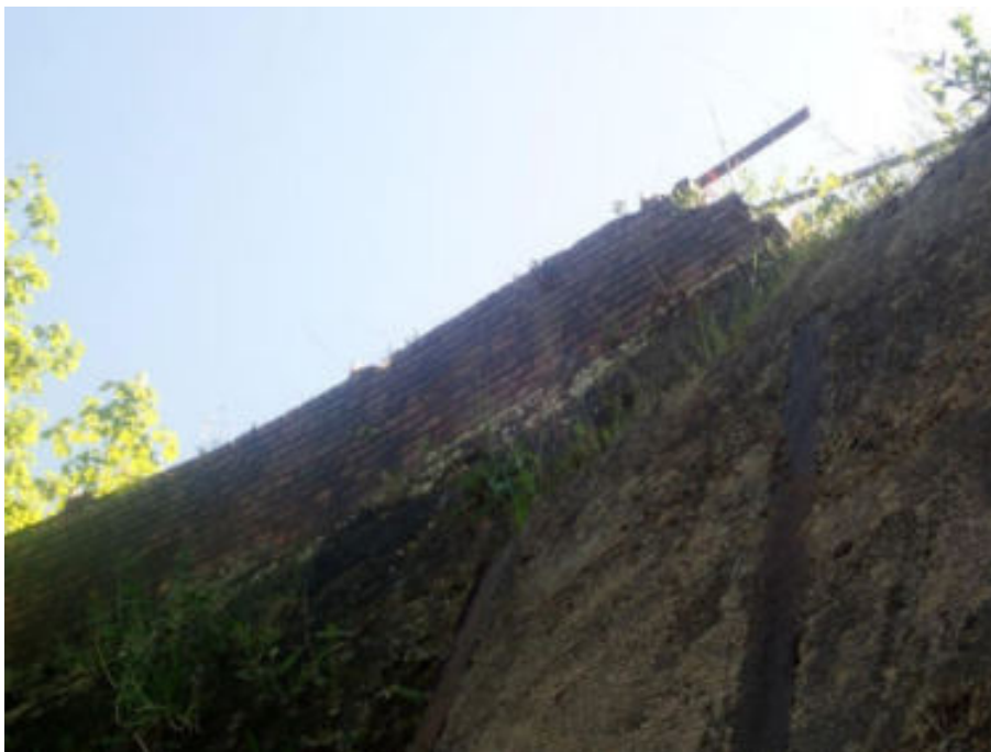
Figure 127. Missing masonry
