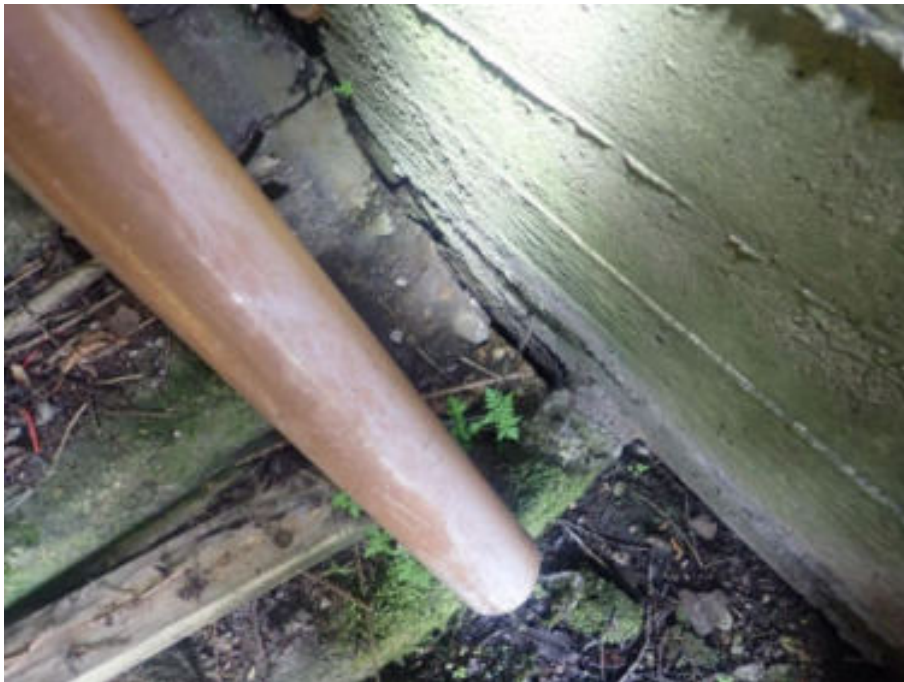
Figure 195. Pipe discharging onto ground
