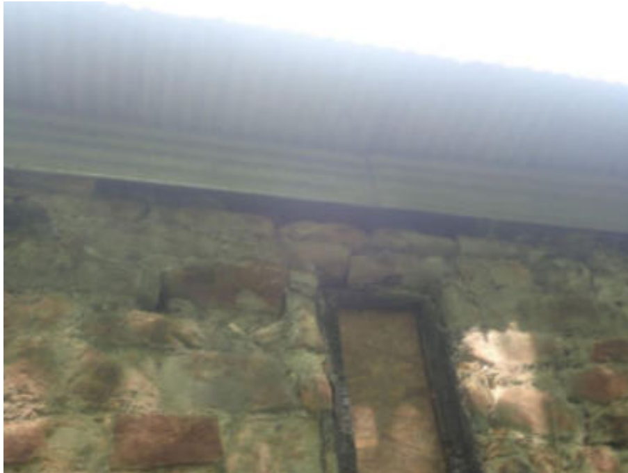
Figure 32. Removed eaves member
