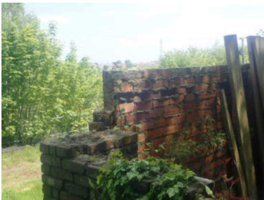
Figure 21. Loose and dislodged panel
