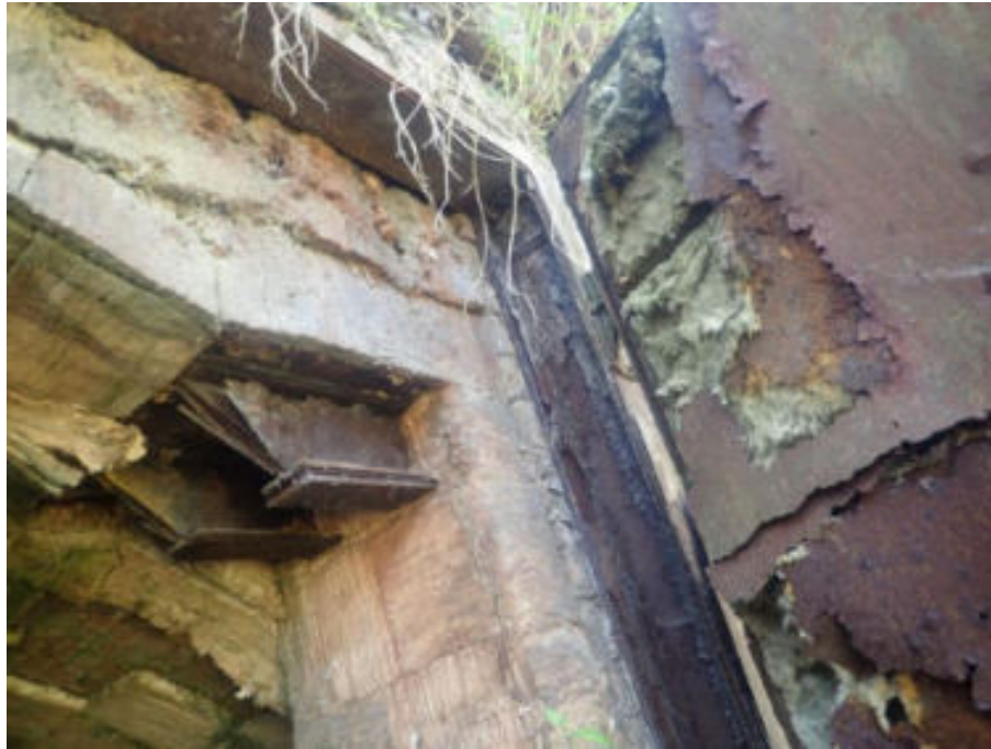
Figure 203. Corroded beam
