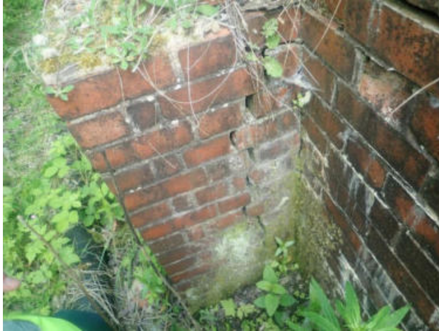
Figure 103. Vertical crack
