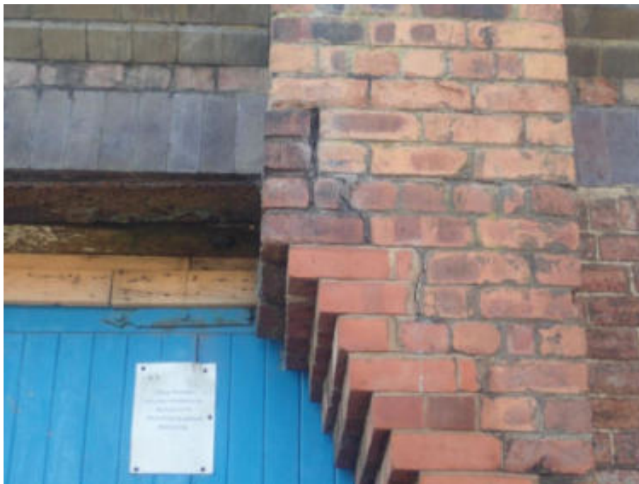
Figure 50. Failed corbel
