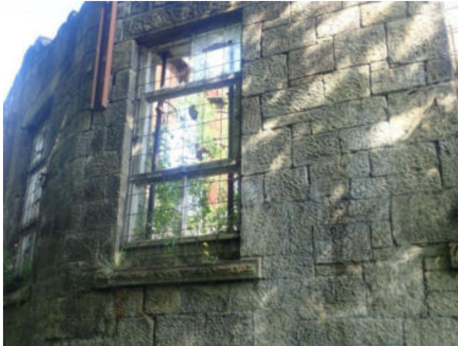
Figure 60. Typical propped lintel
