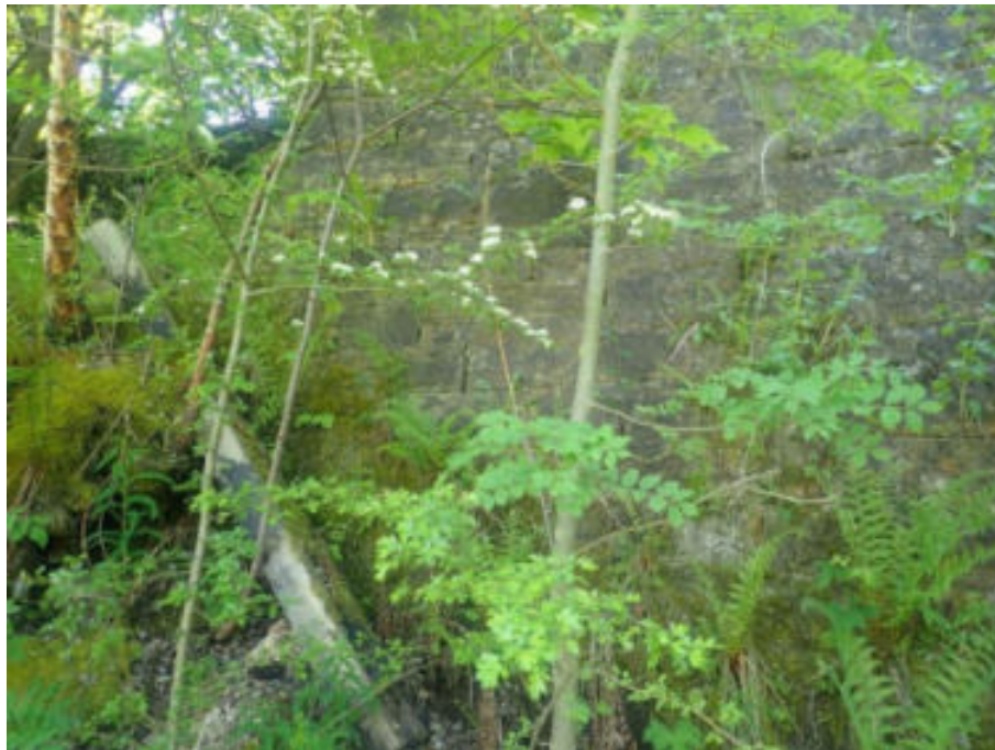
Figure 125. Typical mortar loss
