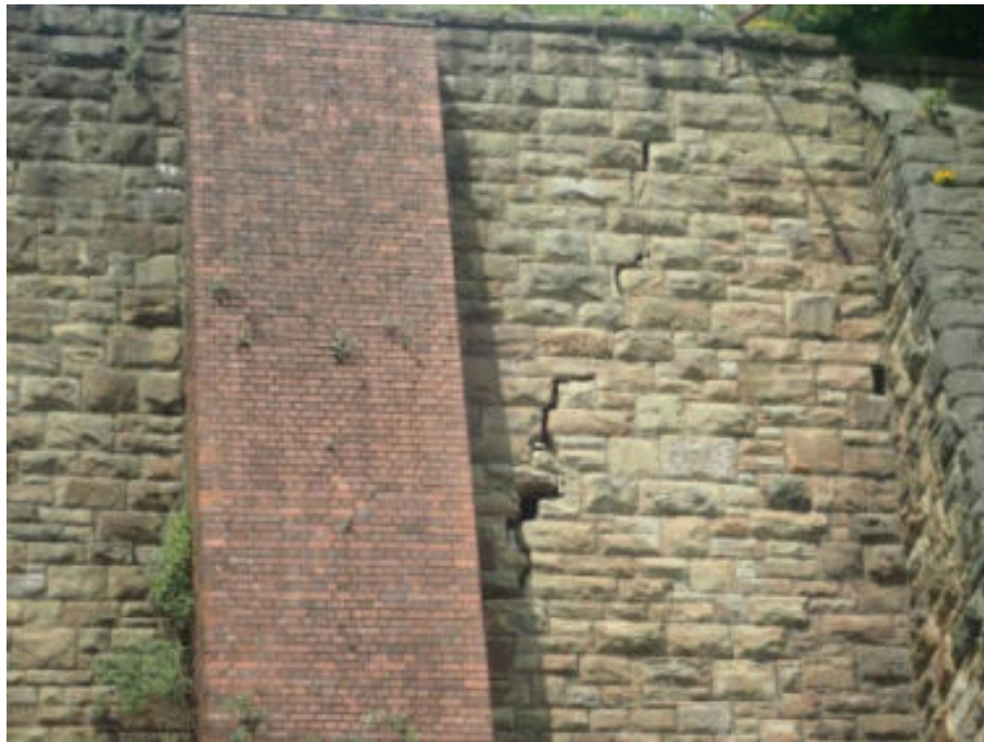
Figure 174. Typical fracture
