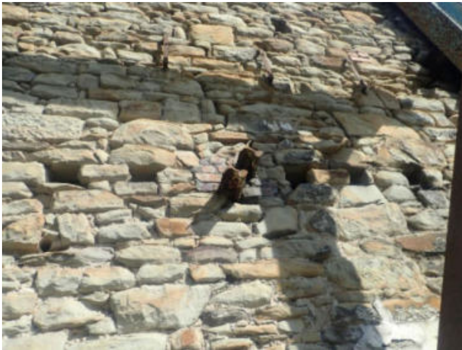
Figure 140. Typical corrosion to steel
