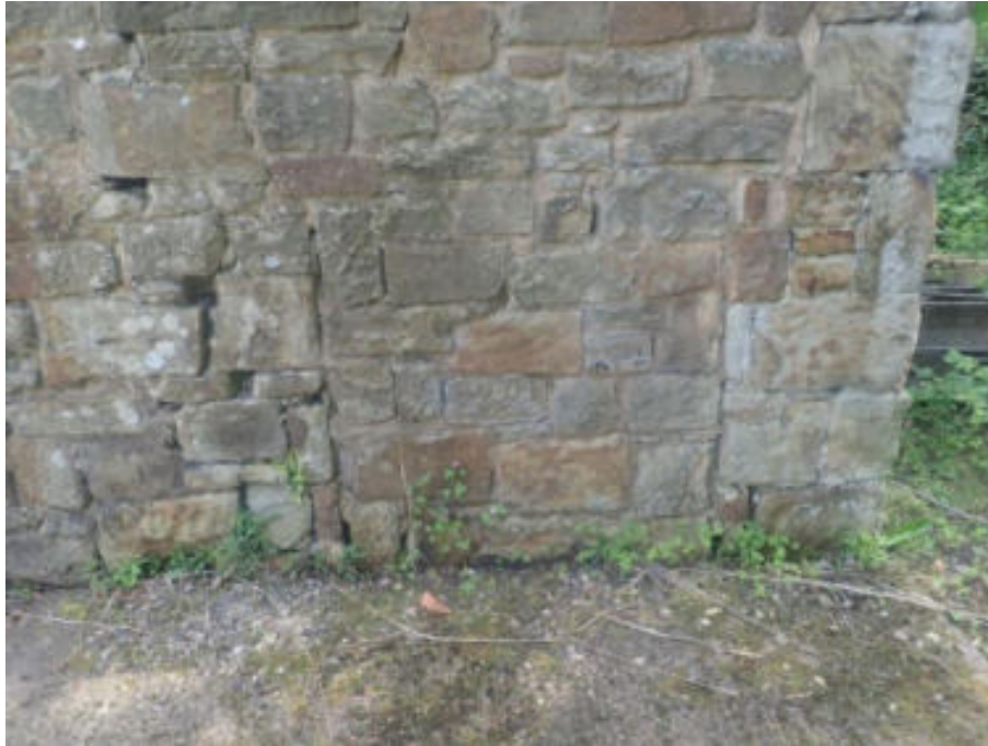
Figure 30. Loose masonry
