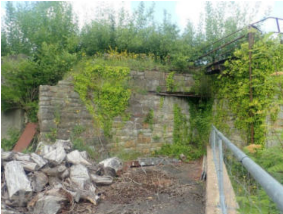
Figure 172. Corroded fence
