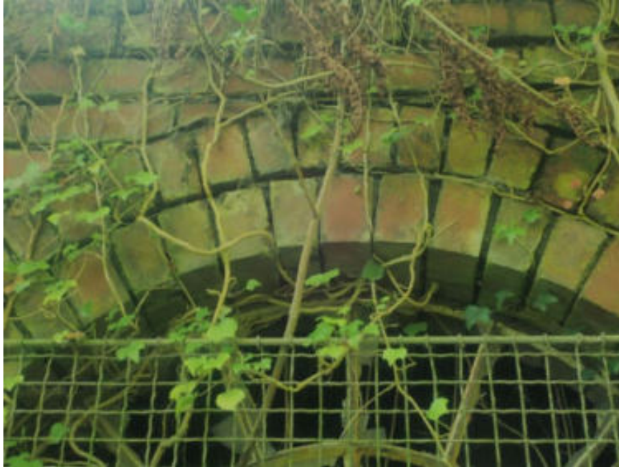
Figure 10. Displaced arch keystone
