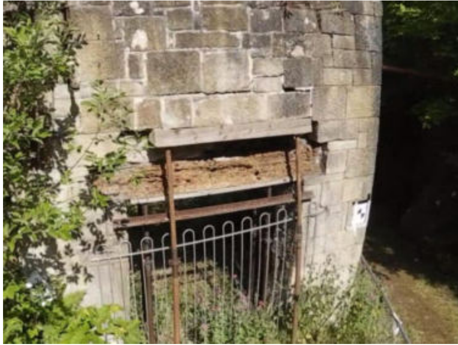
Figure 66. Failed lintel
