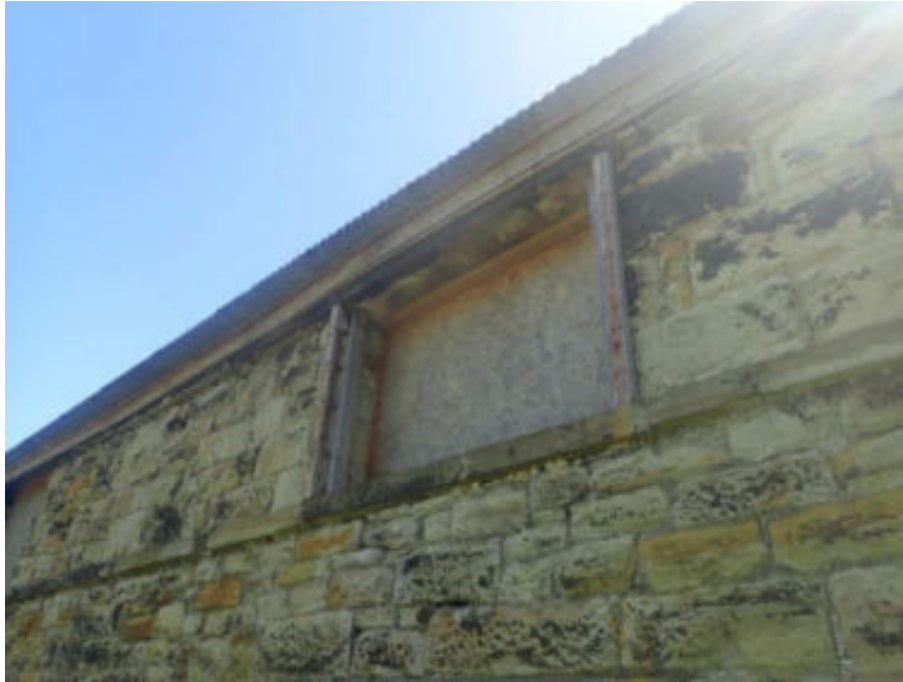
Figure 26. Propped stone eaves beam
