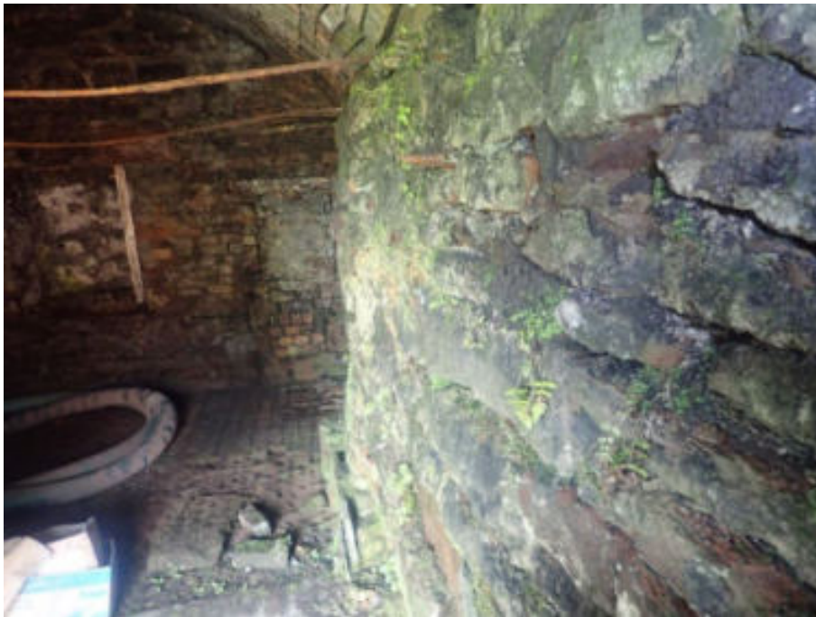
Figure 185. General view of wall
