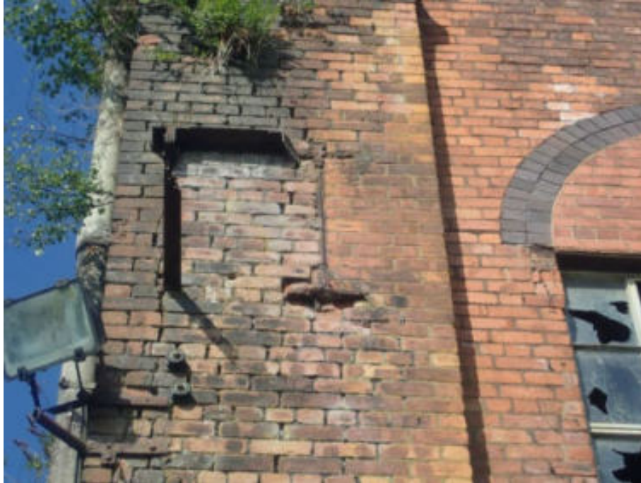
Figure 53. Corrosion to crane beam
