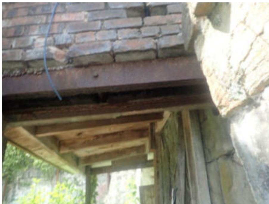
Figure 150. General view of temporary mezzanine
