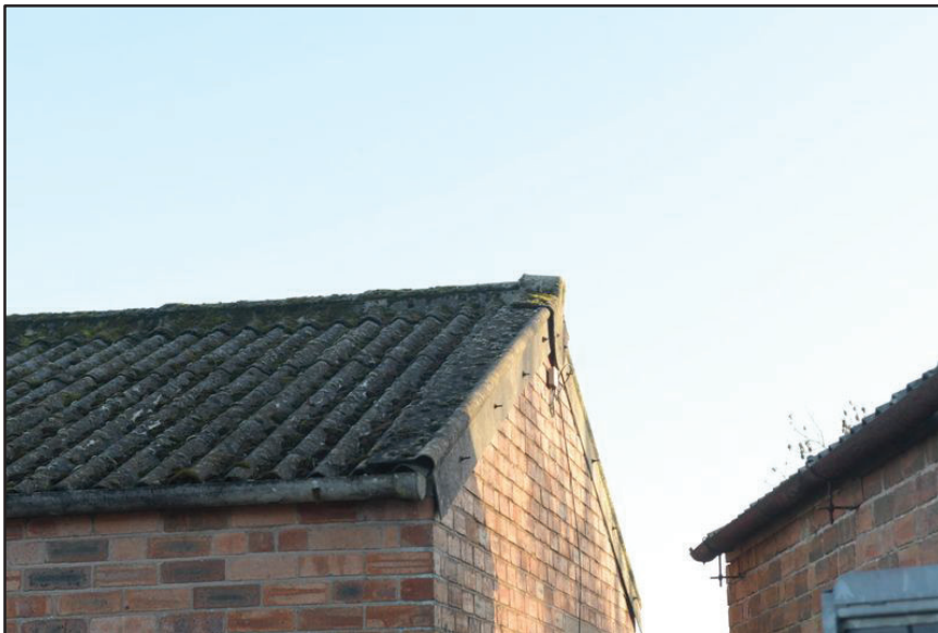
Asbestos end capping
