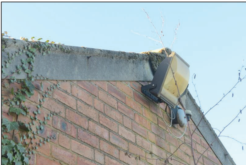
Asbestos end capping
