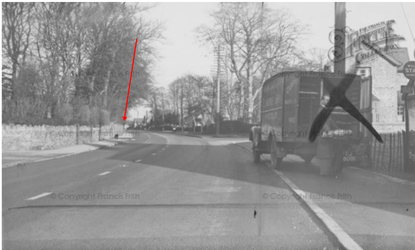
Fig 2. Looking north along Chester Road to The Forks Road c1950. Note the stone boundary to the Golden Lion, which continues along the back of pavement line to meet the brick wall fronting the site at Tyn-y-Coed (arrowed red). (Copyright: Francis Frith).
