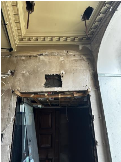
Fig.8 – current stripped out interior
