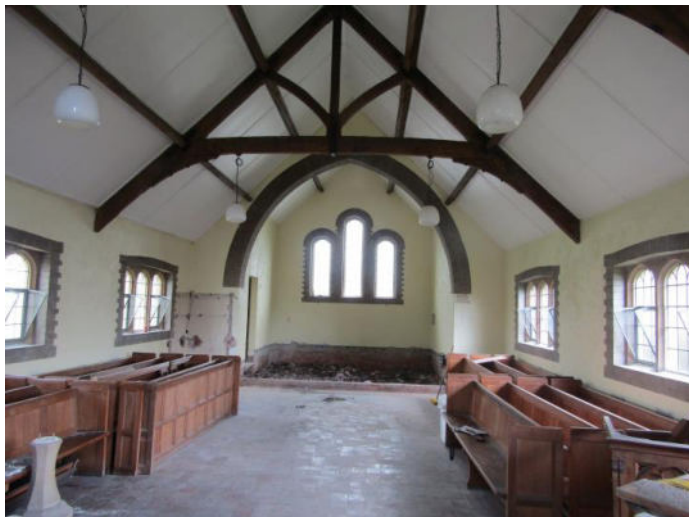
Photo 4: High level of natural light inside building.
