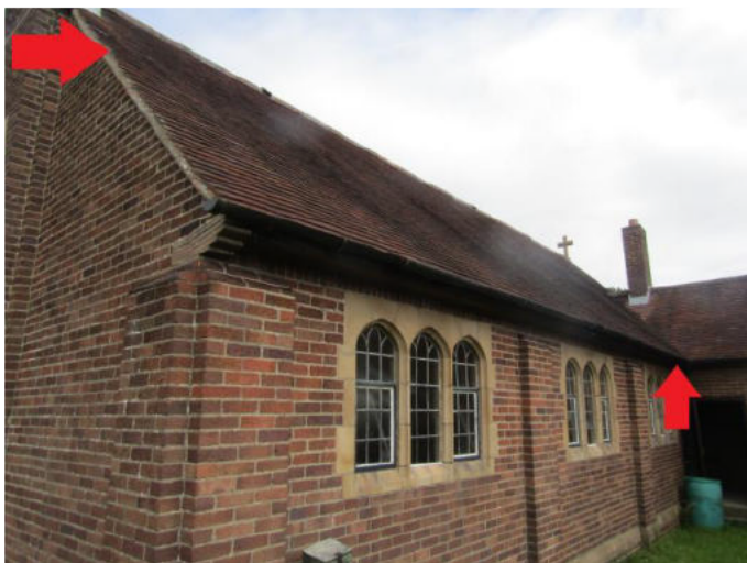
Photo 3: South elevation of former church [red = Common Pipistrelle roost access points].
