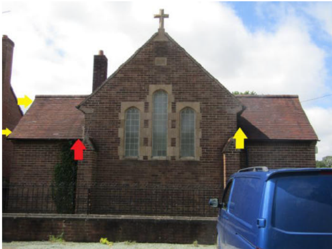
Photo 1: East elevation of former church showing roost access points [red = Common Pipistrelle, yellow = Soprano Pipistrelle].
