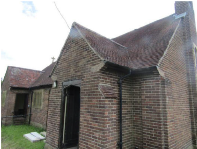
Photo 2: North elevation of former church.
