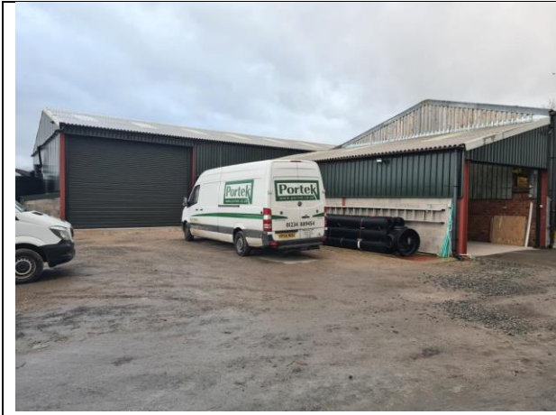
The site. Lean-to removed and replaced.
