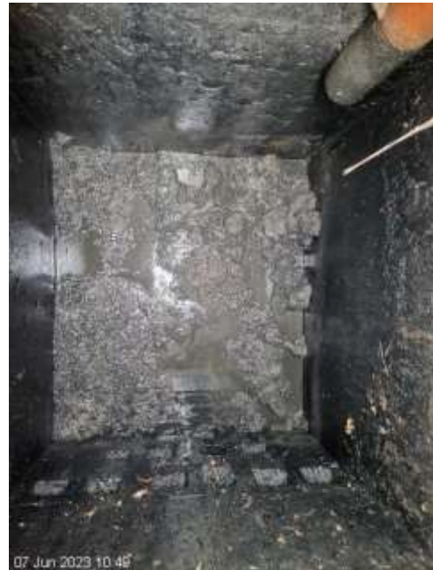
Septic tank After Emptying
