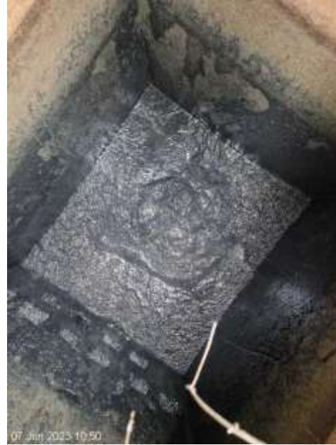
Final Effluent Tank After Emptying
