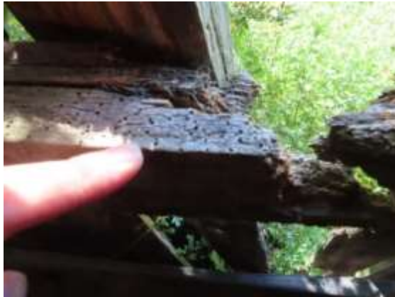
Evidence of wood boring beetle attack
