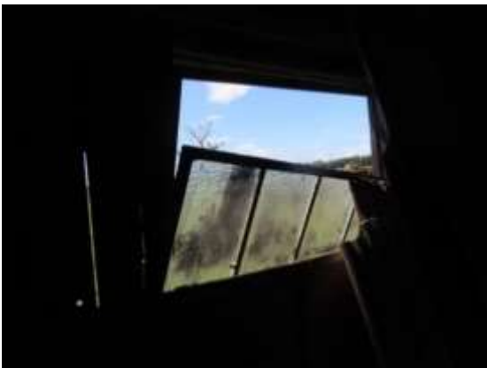
Metal framed window disconnected from frame
