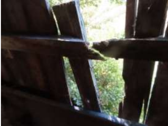
Areas of timber decay to rear elevation frame
