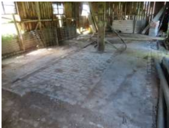
Mixture of brick and concrete floor
