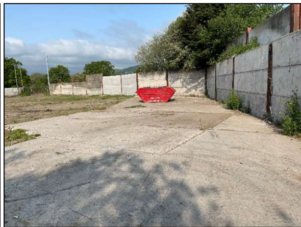
Figure 4: Looking across the area of concrete.
