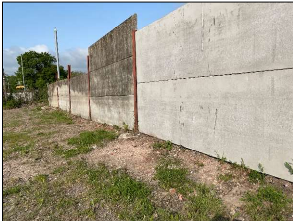
Figure 7: Concrete walls along the site boundaries.
