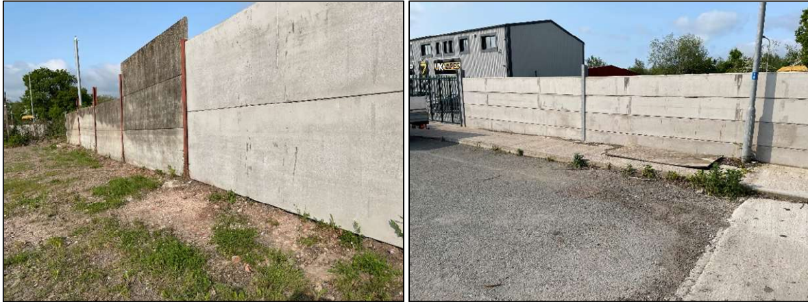
Figure 12: Concrete walls along the site boundaries. Figure 13: Further concrete walls to the south of Miners Road.
