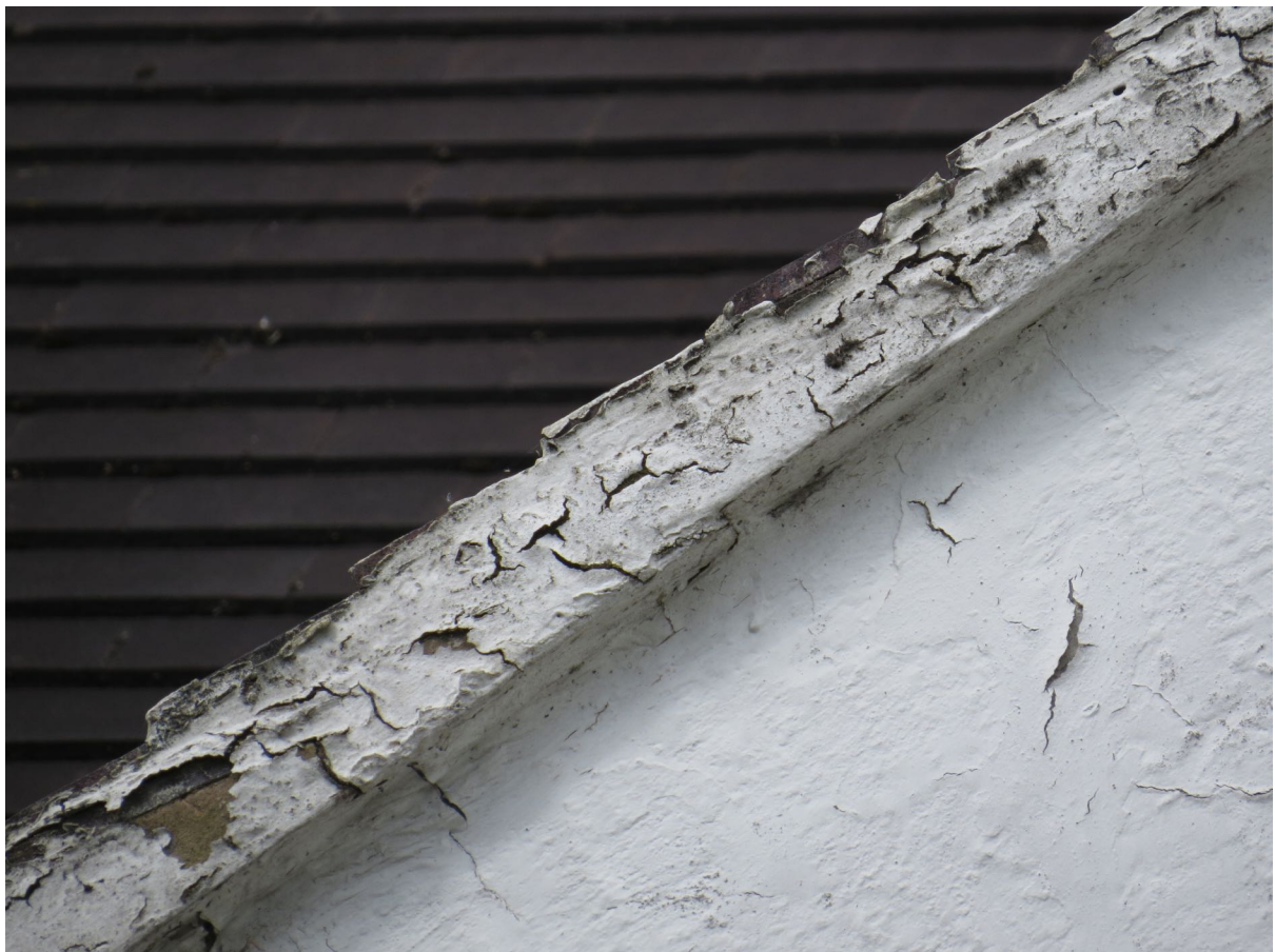
6 – Cement at the gable end verges is intact, with no suitable gaps.
