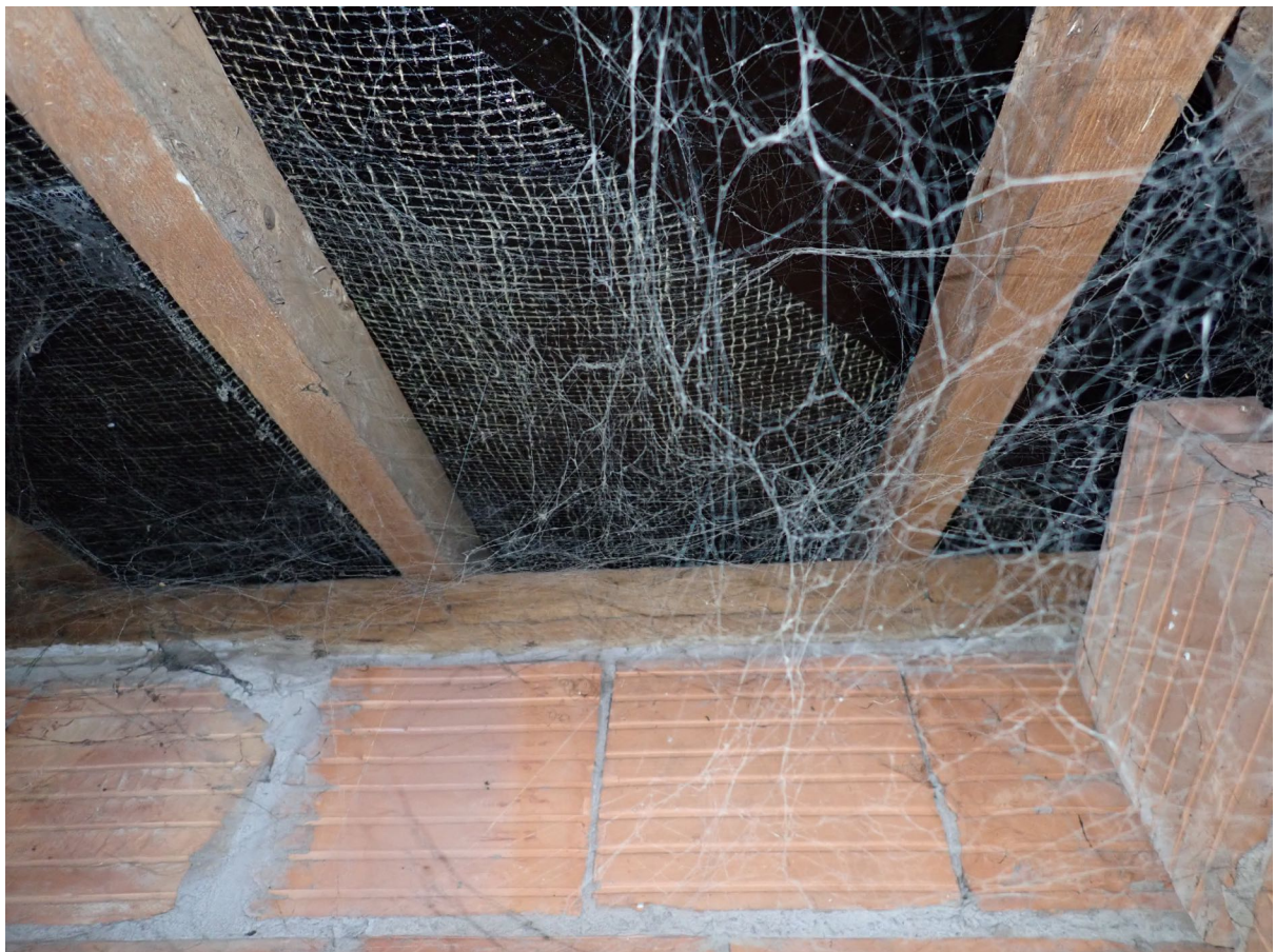
10 – Roof lining is in good condition timbers are covered in cobwebs.
