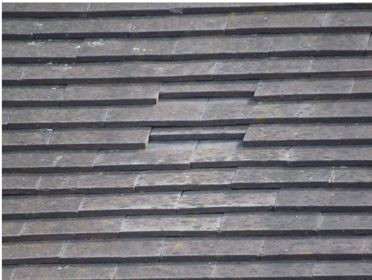
4 – Two slipped tiles at the front of the house do not provide access for roosting bats.
