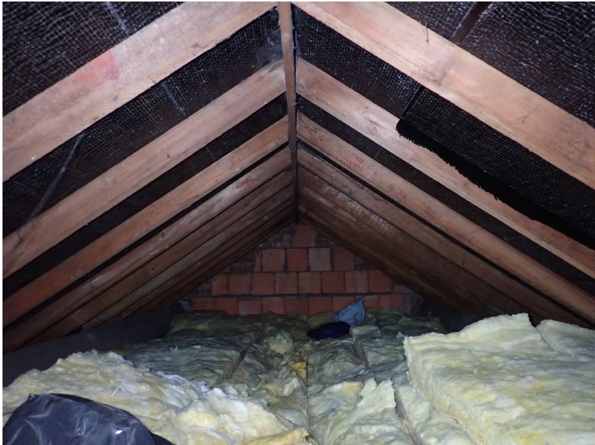
3.2a – The roof void.
