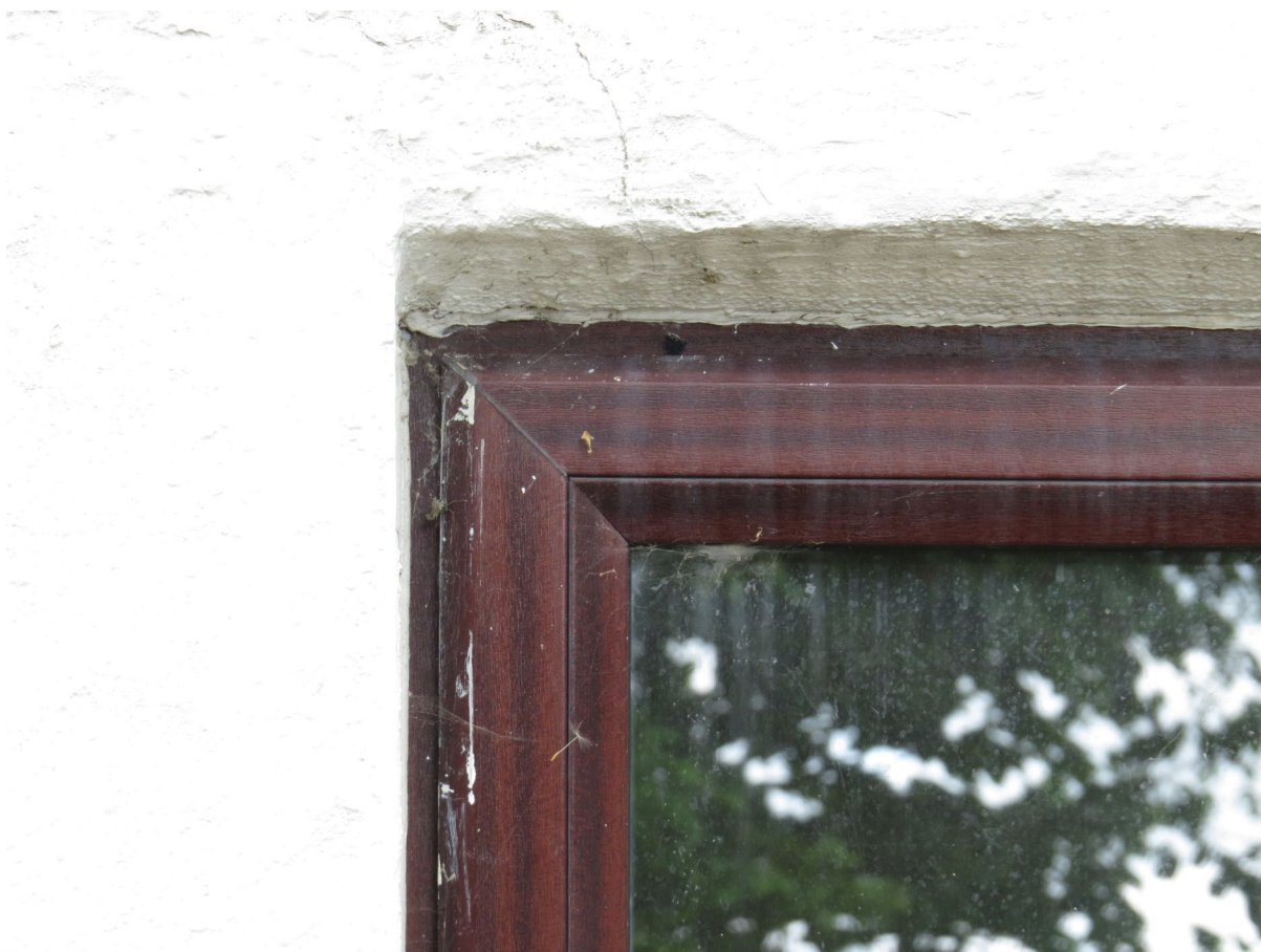
8 – Window and door frames are tightly sealed into brickwork with no suitable gaps.
