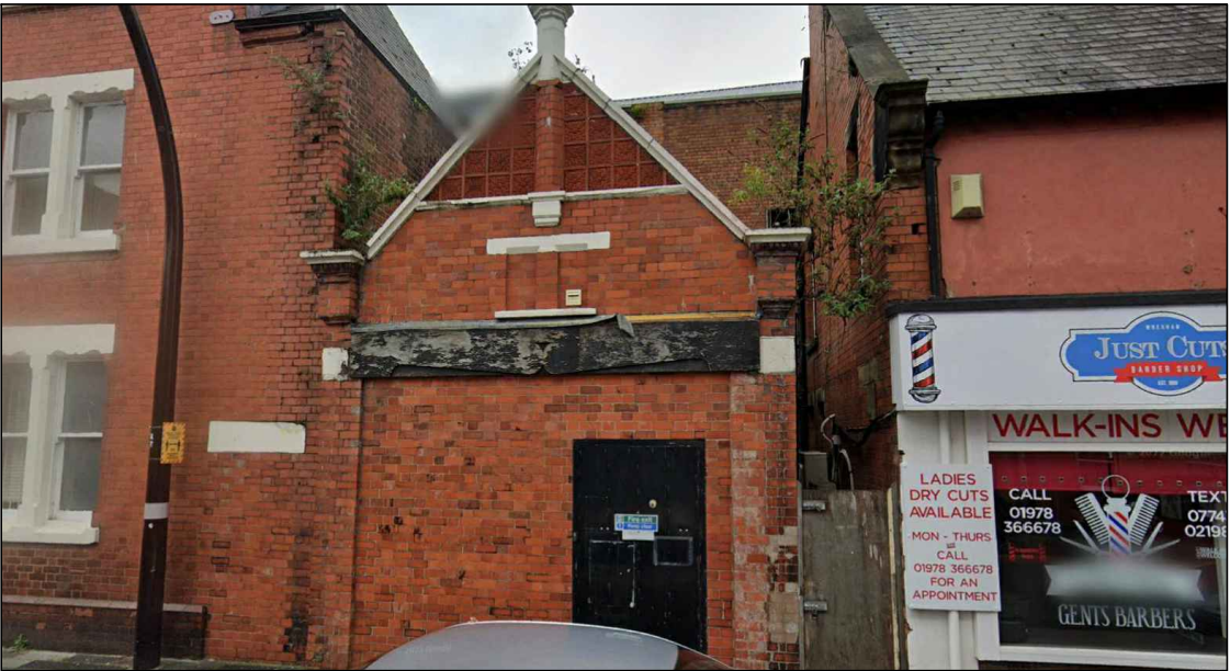
Existing side rear access photo
