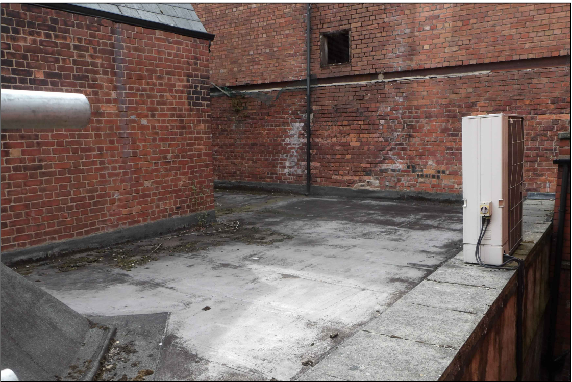
Existing flat roof photo
