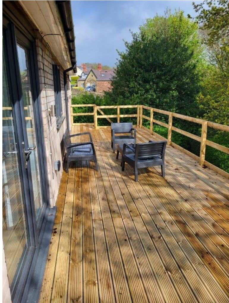
Image 1 - looking north west towards neighbouring property n.25, illustrating the significant intervening distance and potential for acceptable mitigation measures
