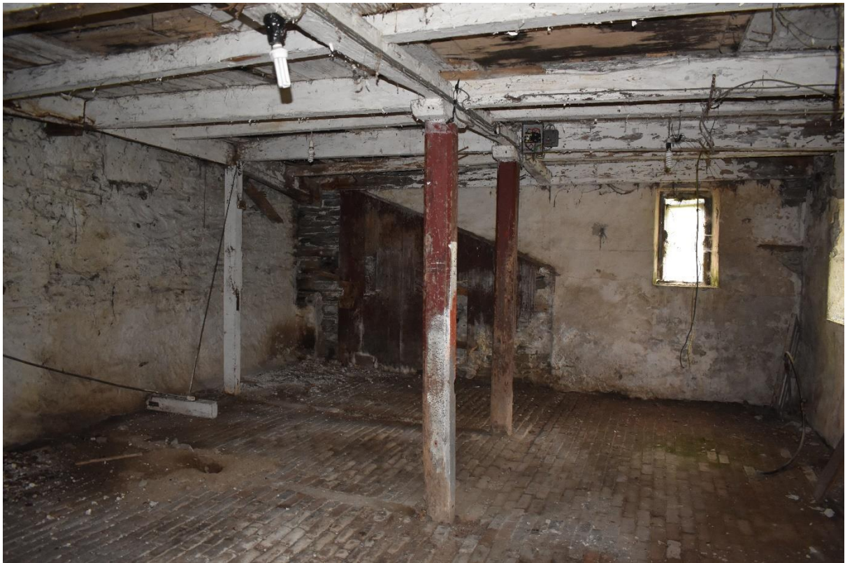
Figure 3.9: The larger of the two ground floor rooms, within the far wall of which one of the wren nests was found.
