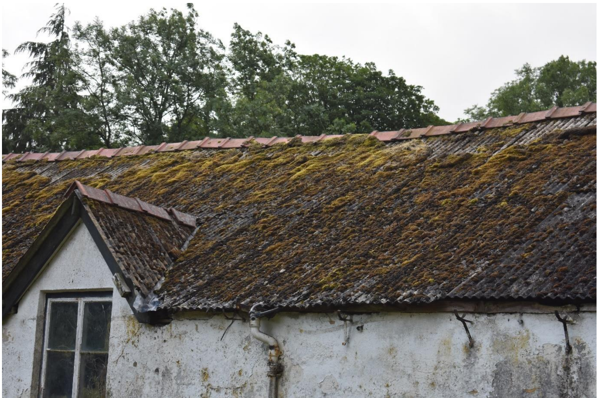
Figure 3.5: The condition of the front roof and roofline.
