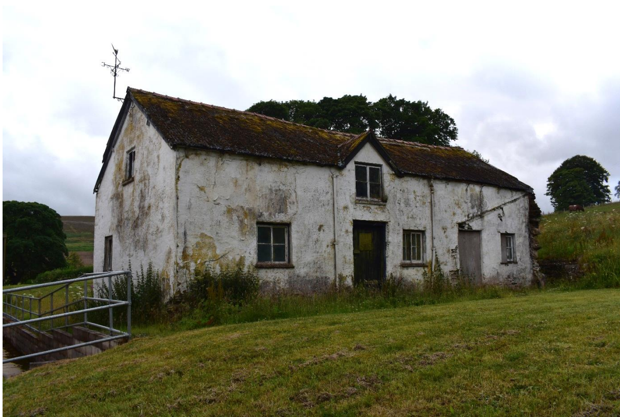
Figure 3.2: The north-facing (front) elevation and east-facing gable of the building.
