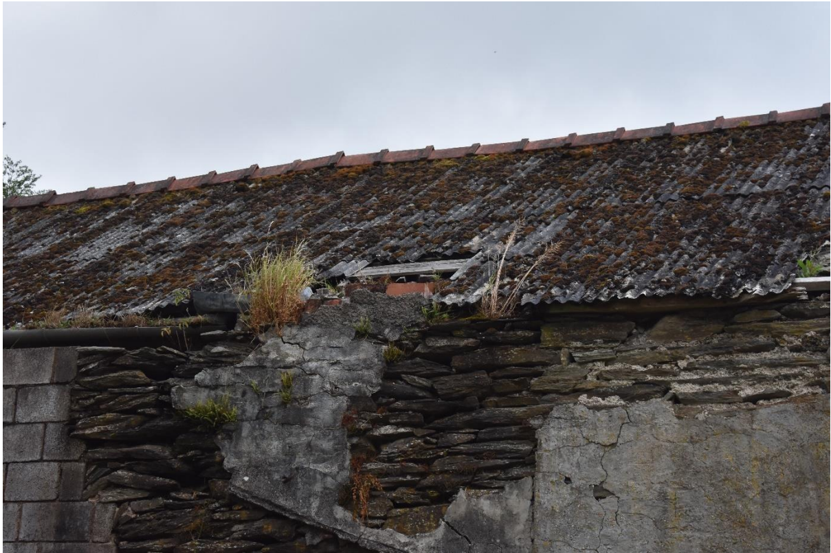
Figure 3.6: The condition of the rear roof and roofline.
