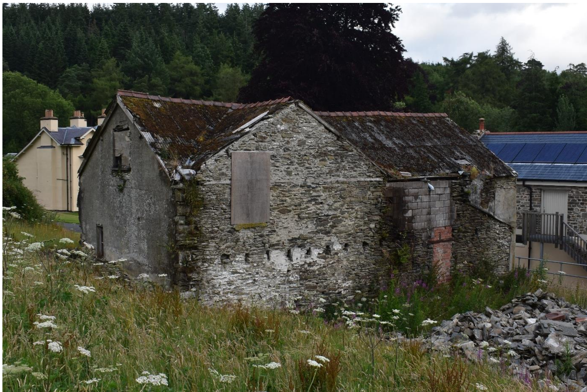
Figure 3.3: The south-facing (rear) elevation and west-facing gable of the building.
