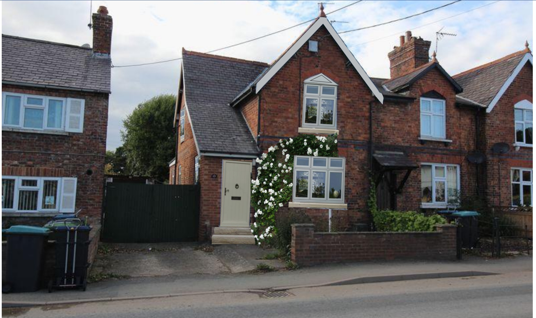
Plus additional replacement of stone window sills to match historic sills (see adjoining property).
