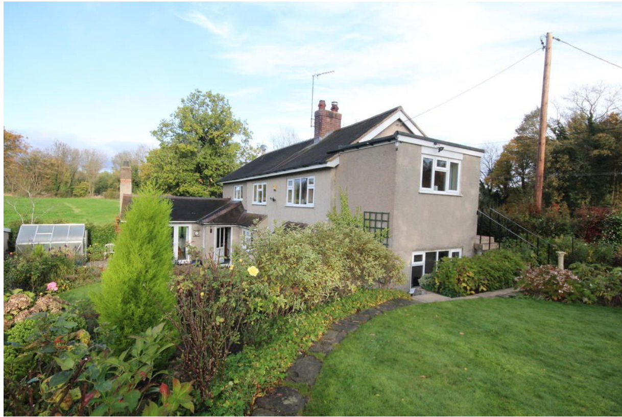
Modern two storey flat roofed extension to the south is out of character. Proposals to demolish down to first floor slab for new roof terrace.
