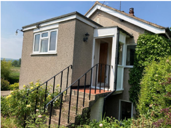
Existing overlooking from dressing room, bedroom and stair
