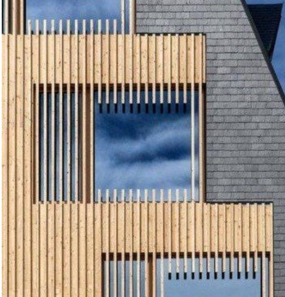
Fins projecting outwards and extending upwards from boarded backing panels. Larch in early stage of weathering
