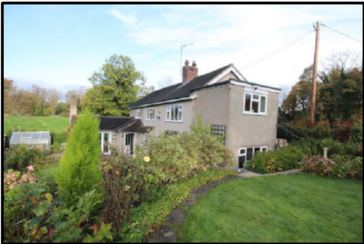
As existing (view North)
