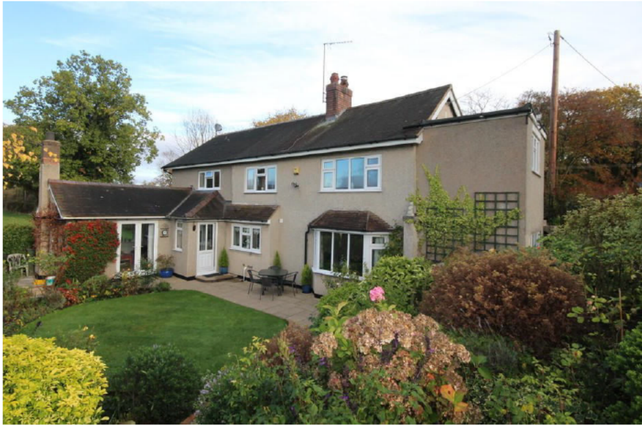
Existing garden elevations. Modern 2 storey extension on right side
