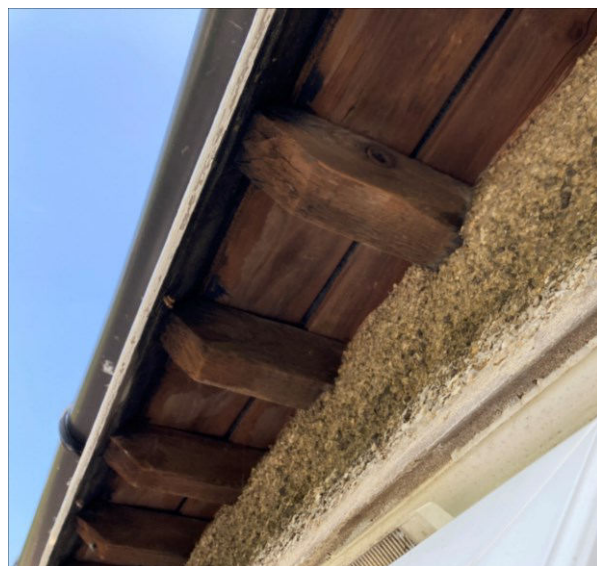
Existing house eaves detail: timber structure projecting from the boards
