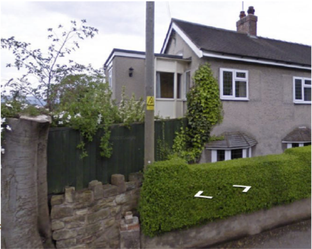
Drws-y-Coed viewed from road, dressing room visible
