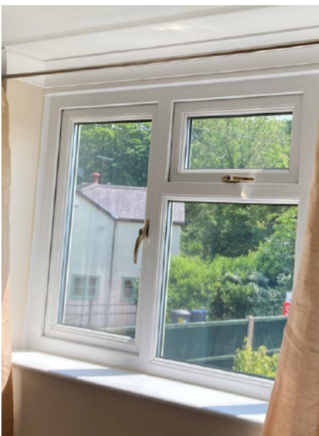
Foundry House – Viewed from 1 st floor dressing room window
