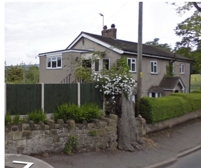
Out of character modern first floor extension to be demolished
