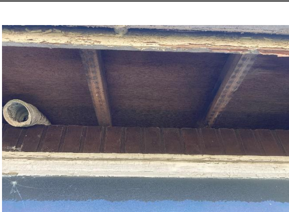
Plate 5: The gaps between the open rafters allowing direct flight access into the loft space across the front of the building
