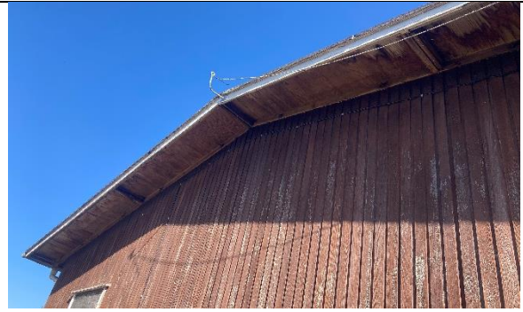
Plate 2: The well-sealed gable ends of the building. No PRF's present.
