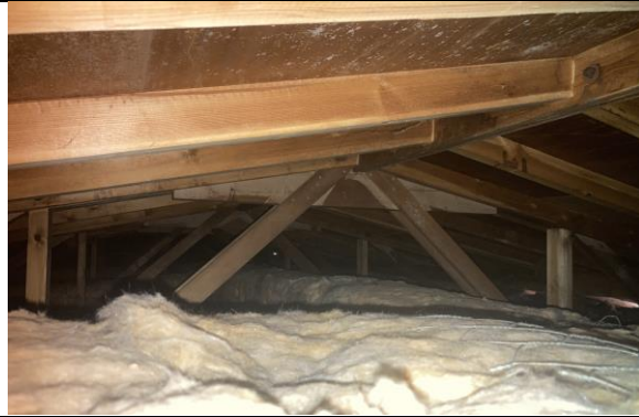
Plate 6: loft space, 750mm height 'clean' timber framing
