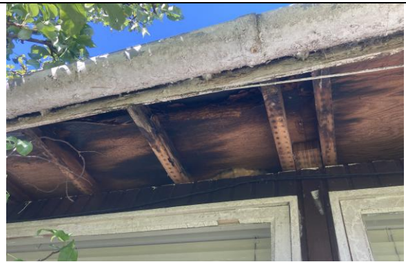
Plate 4: The gaps between the open rafters allowing direct flight access into the loft space across the front of the building.
