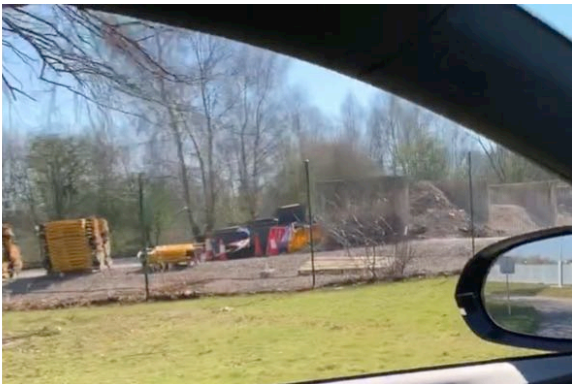
View of open storage bunker walls
