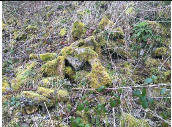
8. Stone rubbles of an old shed existing in the central part of the site.
