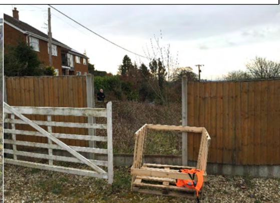
4. Temporary access to the site through a wooden hoarding from the north.
