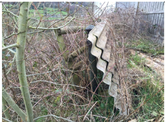
12. Fibre cement roofing sheet used as provisional hoarding on the northern boundary.
