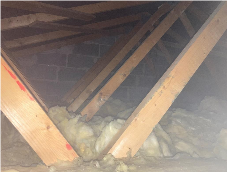
A.1.9 Plate 9: Internal roof structure of B2
