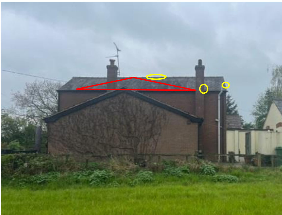
A1.6 Plate 6: Building B1 potential roost features shown and area of slates to be removed (red)
