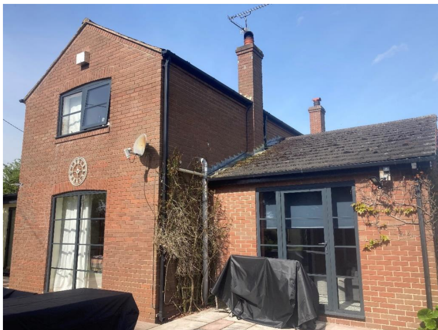
A1.3 Plate 3: View of the eastern aspect showing Building B1 and B2
