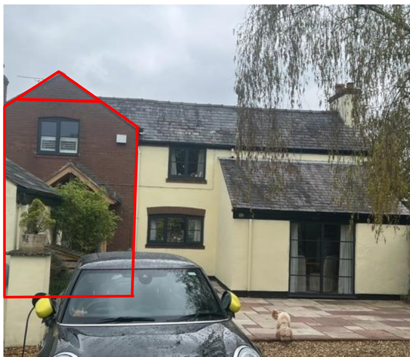
A1.2 Plate 2: View of the northern aspect showing single storey extension (B2) and two storey brick extension (B1)
