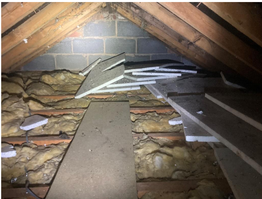
A1.7 Plate 7: internal roof structure of B1
