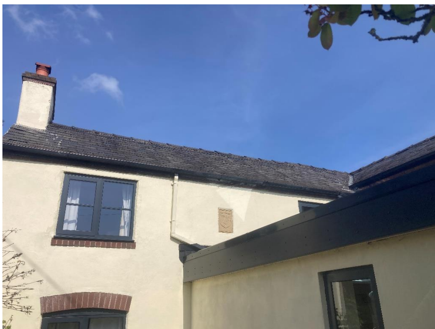
A1.4 Plate 4: Showing eastern aspect of the original cottage, roof in good condition.
