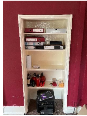
Door opening to be reinstated.
