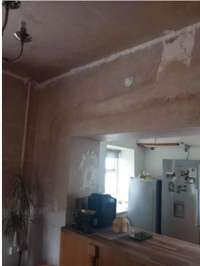
7. Kitchen wall to be uplifted to ceiling height
