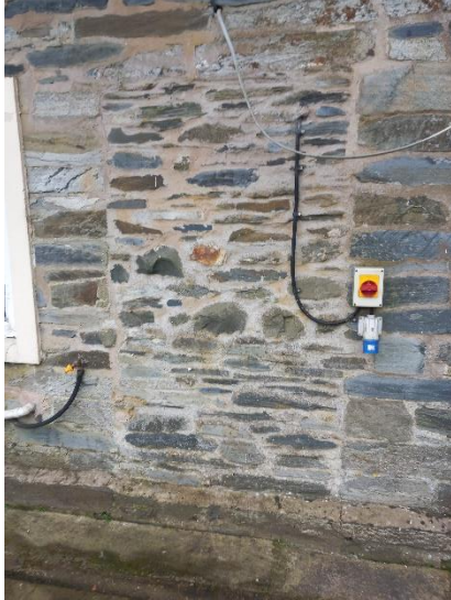
6. Original doorway from kitchen to outdoors
